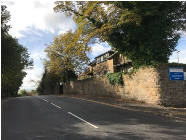
1. View of the site looking up Mount Vernon Road.
