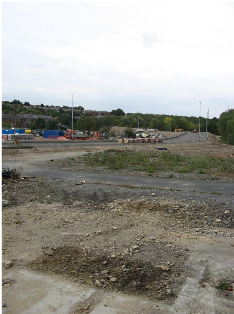
Plate 4: Showing the new road construction on the Northern Site
