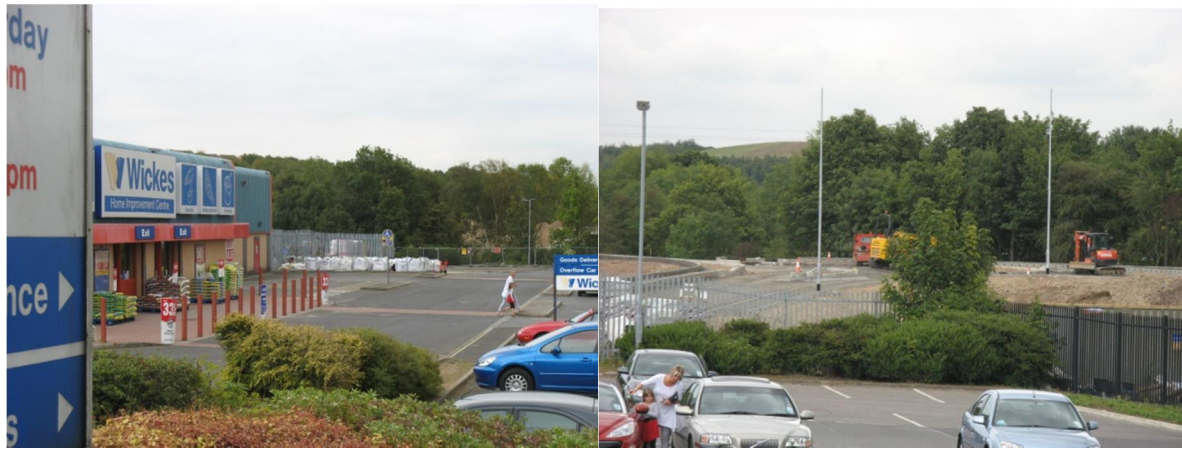
Plate 3: Showing the Commerical Unit and Adacent works for the new road being built on the former gasworks (Northern Site)
