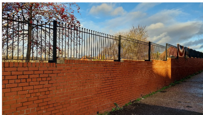
Photograph 12: Red brick wall and metal railing forming the southern boundary of the site.
