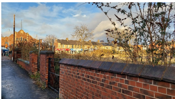
Photograph 11: Western boundary (photograph taken from High Street) showing the red brick wall and scrub immediately adjacent to and within the red line boundary.
