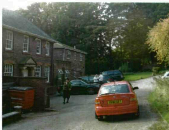
The front of existing Bollinbroke House Care Home and its car park
