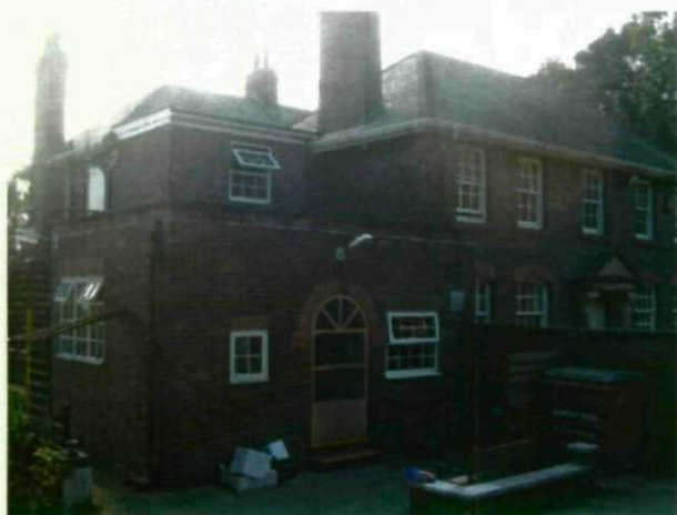
The front of existing Bollinbroke House Care Home
