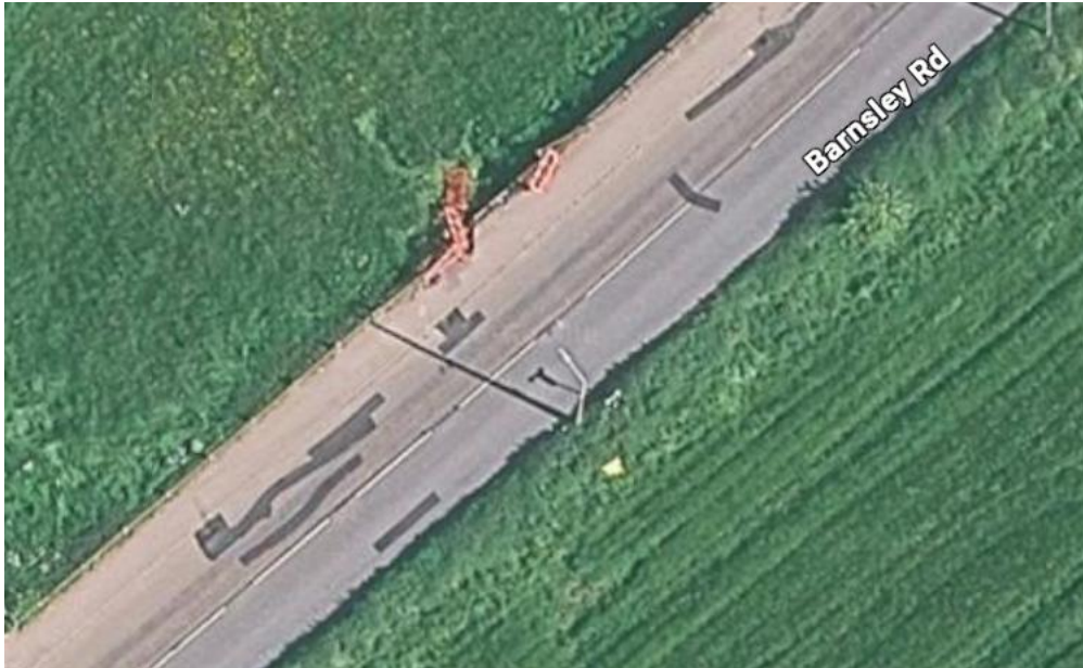
Fig 3 Photograph showing a view of the damaged fencing with temporary safety barrier which has repeatedly been put back in position by the owner of the field
