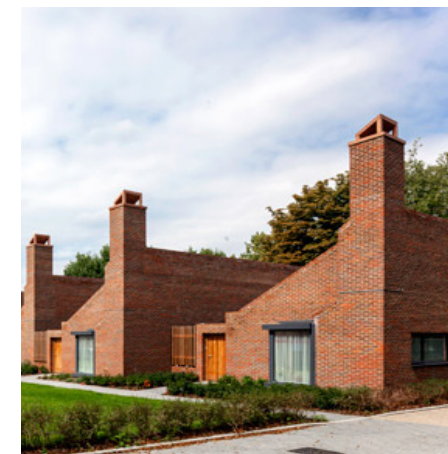
D. Continuous brick gables and wall, with large openings and secure gates
