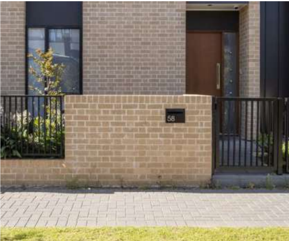
LOW-LEVEL WALLS WITH RAILINGS
