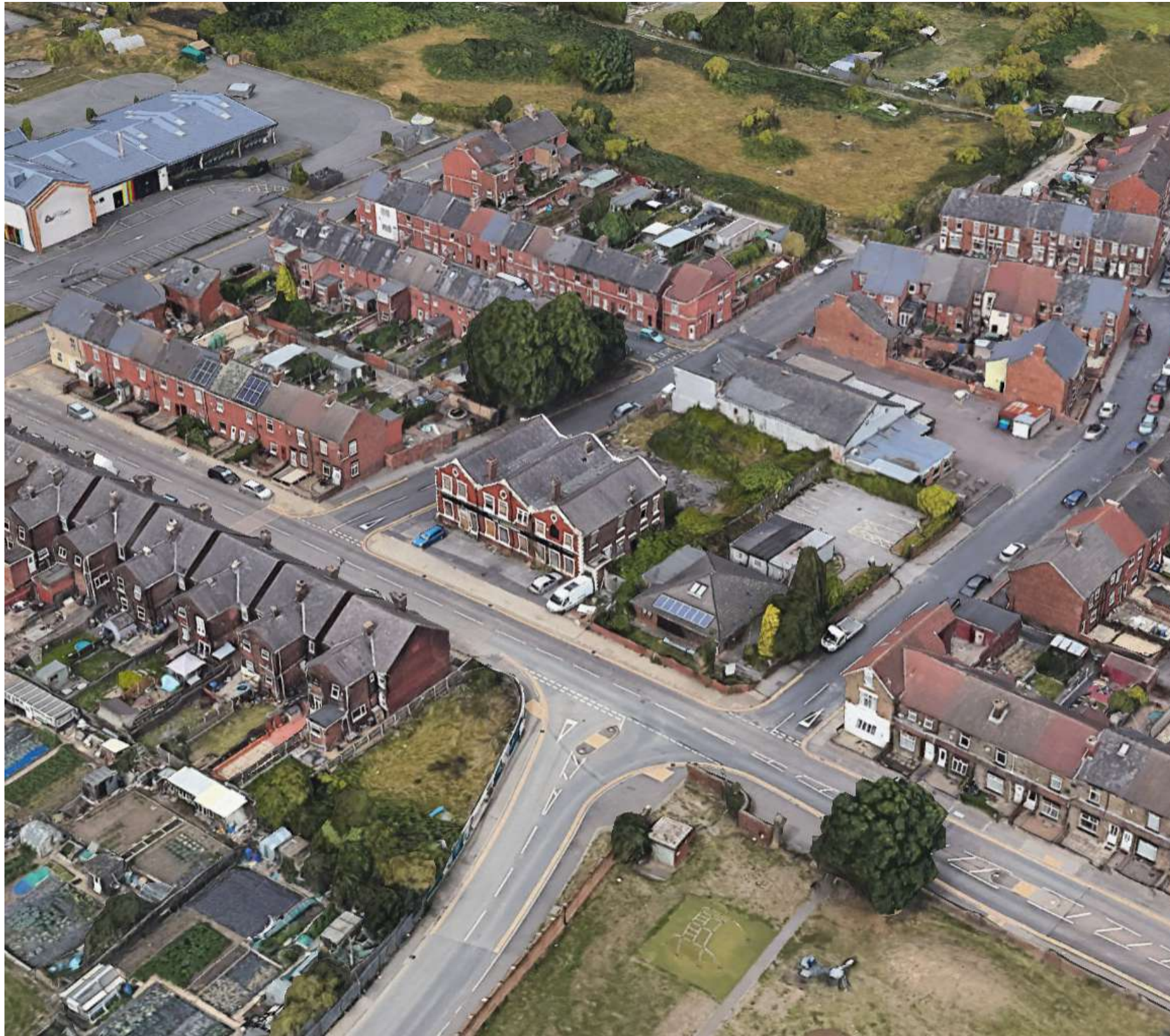
AERIAL VIEW BEFORE DEMOLITION
