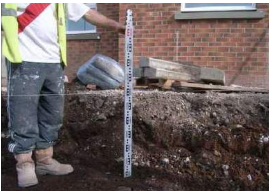
Photograph 5: Depth check of inert cover within rear gardens. Taut string line spans across excavation.
