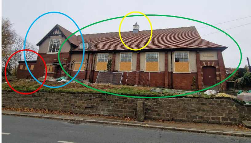
Photo 1. Brierley Village Hall showing the three main sections of building as demarcated by the green, blue and red circles. The central belltower is demarcated by the yellow circle. The areas shown in the green, blue and yellow circles are to remain in-situ, whilst the one-storey extension shown in the red circle is to be demolished as part of the Proposed Development.
