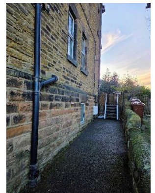
Pathway access to carpark
