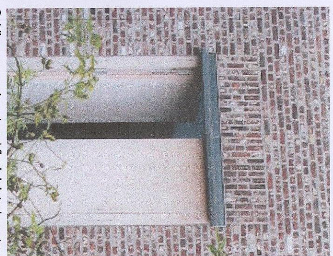
Soldier course band and flush jointed mortar.
