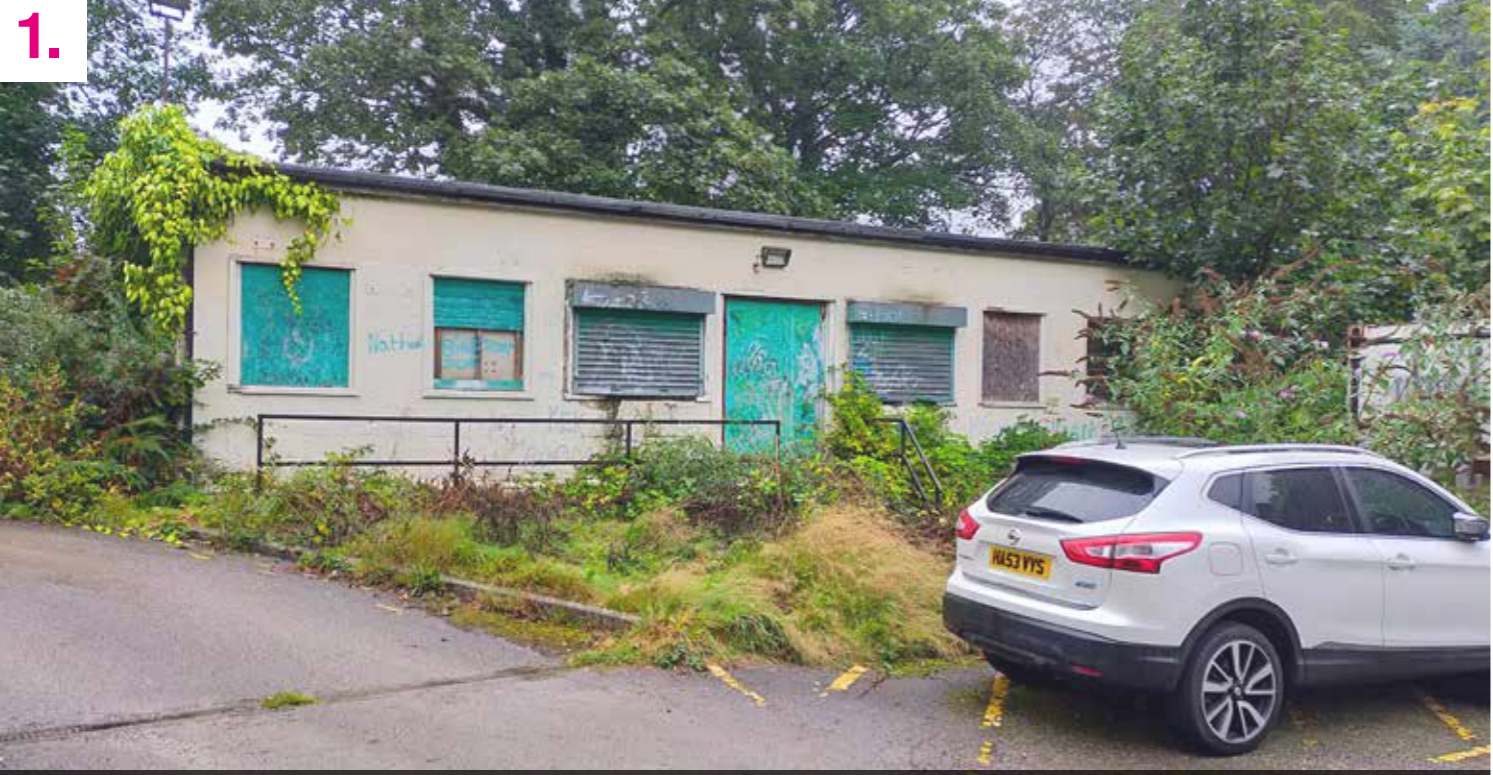
Above: Existing workshop outbuilding, facing north
