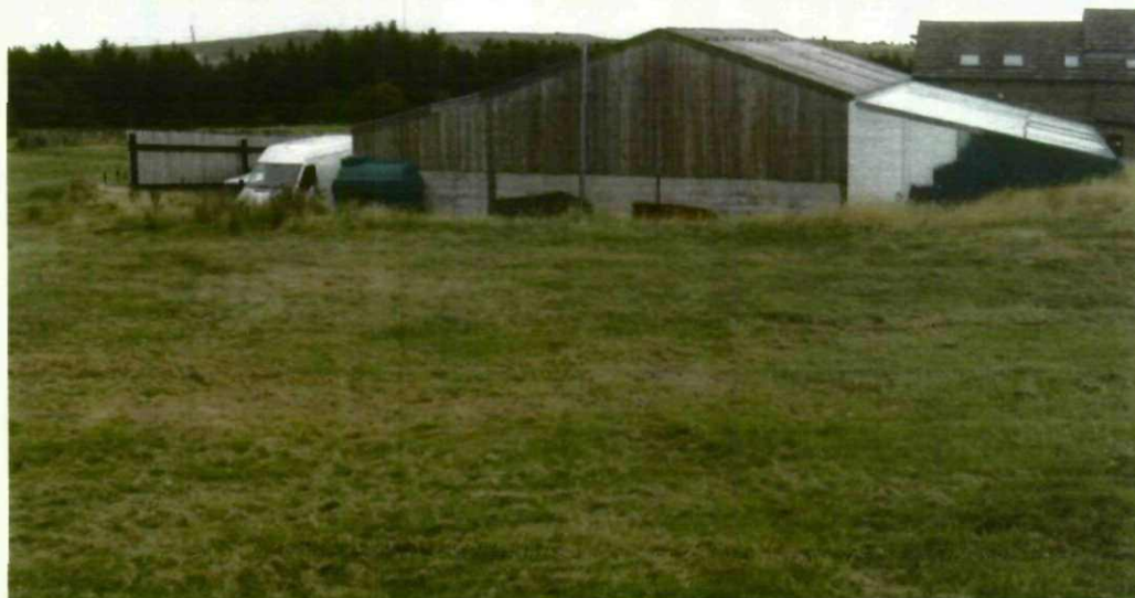
Rear of outbuilding and site of proposed kennel block.
