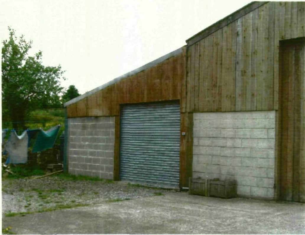
Outbuilding to be converted to hydrotherapy centre.
