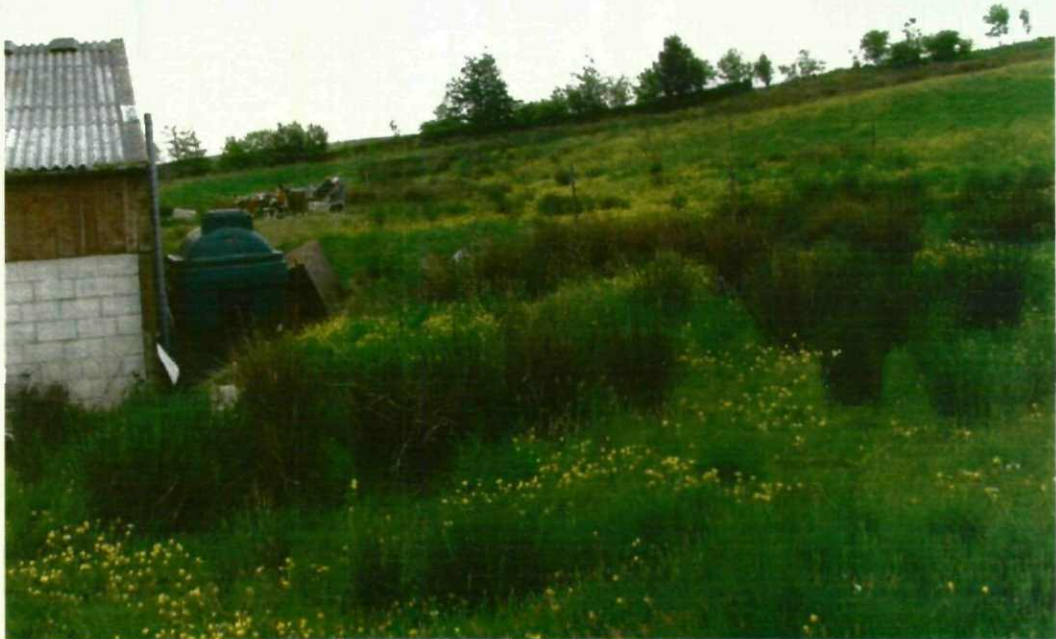
Site of the proposed kennel block; to be built into the bank.
