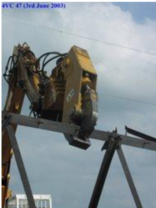
Plate 2.16: Steelwork Breaker and Steelwork Ready for Loading into a Skip
