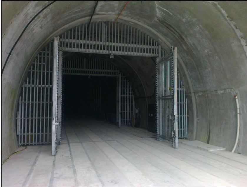
Plate 2.2: Existing Cable Troughs at the Woodhead Tunnel
