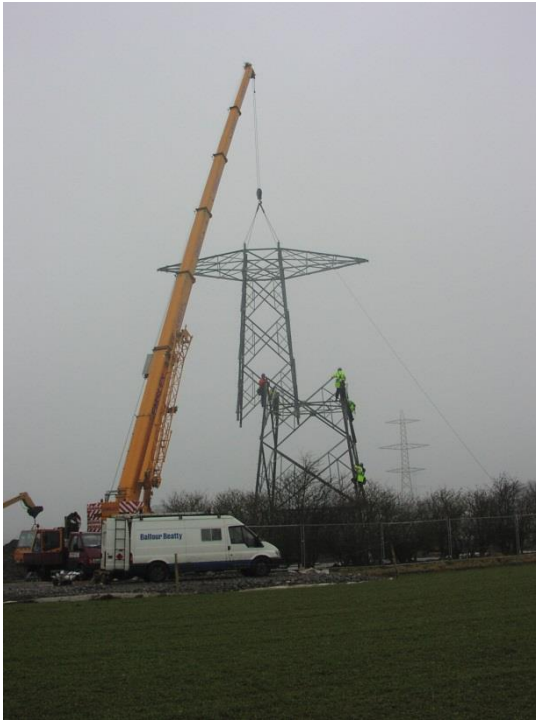
Plate 2.10: Pylon Erection using a Mobile Hydraulic Crane
