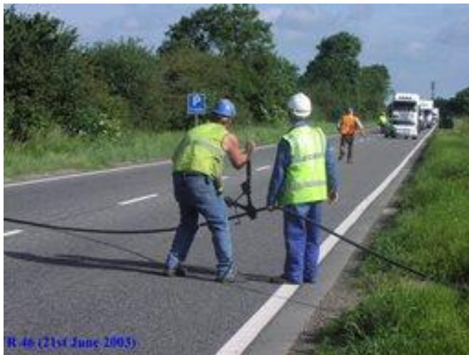
Plate 2.12: Overhead Conductors on Road Ready for Removal
