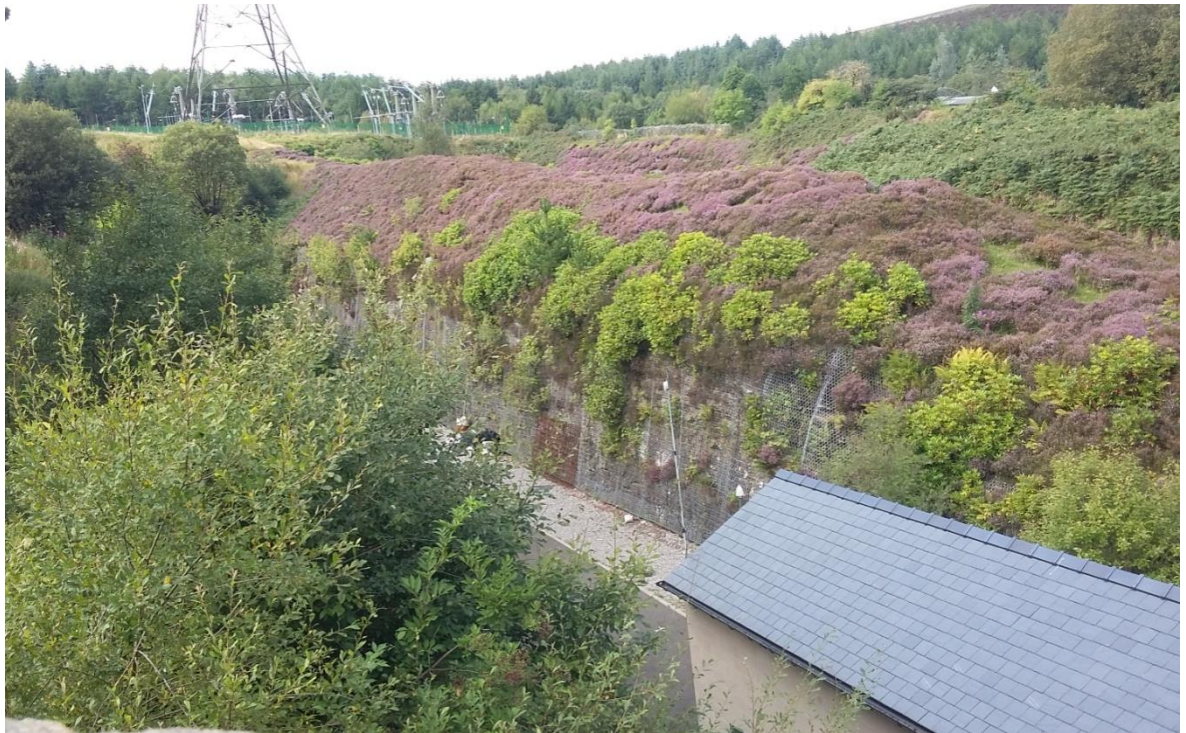
Plate 2.3: Embankment to be partially removed to accommodate Cable Corridor
