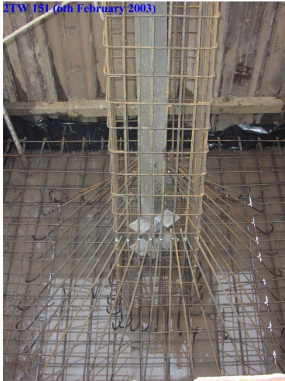
Plate 2.8: Reinforcing bar in place
