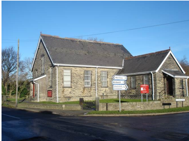
Fig 06. Methodist Chapel opposite site
