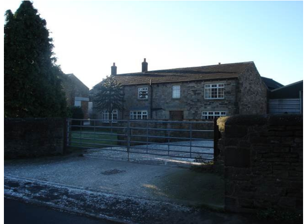
Fig 09. Ivy House Farm – East Elevation
