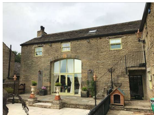
Fig 02. East Elevation of Holly Barn
