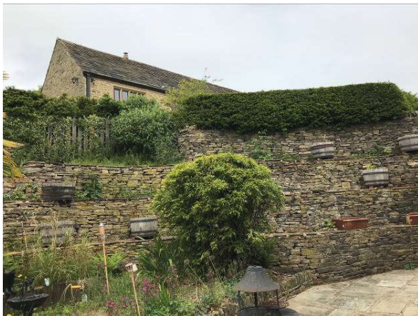
Fig 3 – Grouped photos of rear garden area showing rear (west) elevation of Holly Barn, retaining wall built of terraced dry-stone walling and view of The Court House beyond west boundary.
