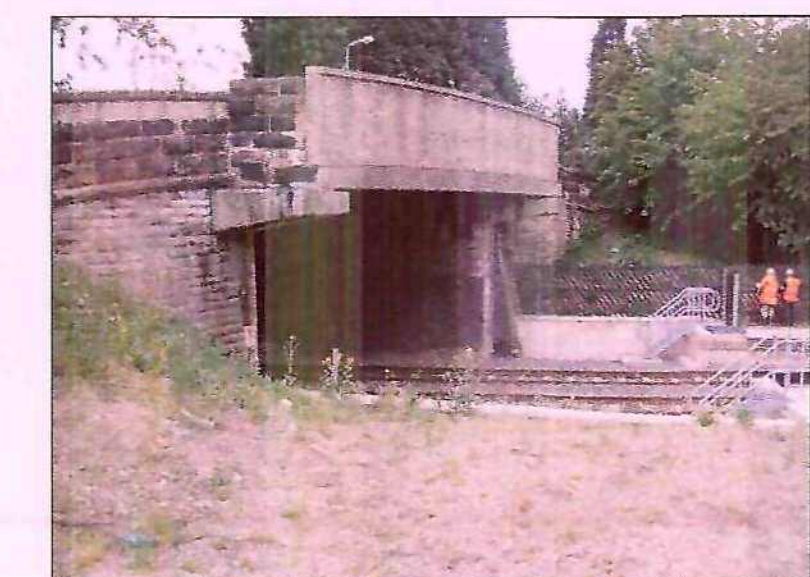
VIEW OF UP PLATFORM, NEAR LOWFIELD ROAD OVERBRIDGE. THIS IS THE PROPOSED PLACE FOR A FOOTBRIDGE
