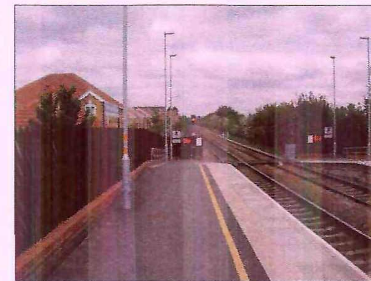
EXISTING FOOT CROSSING. VIEW FROM DOWN PLATFORM
