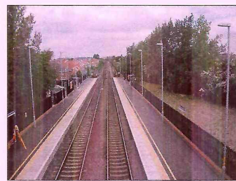
GENERAL VIEW FROM THE ROADBRIDGE LOOKING NORTH, EXISTING CROSSING IN THE BACKGROUND
