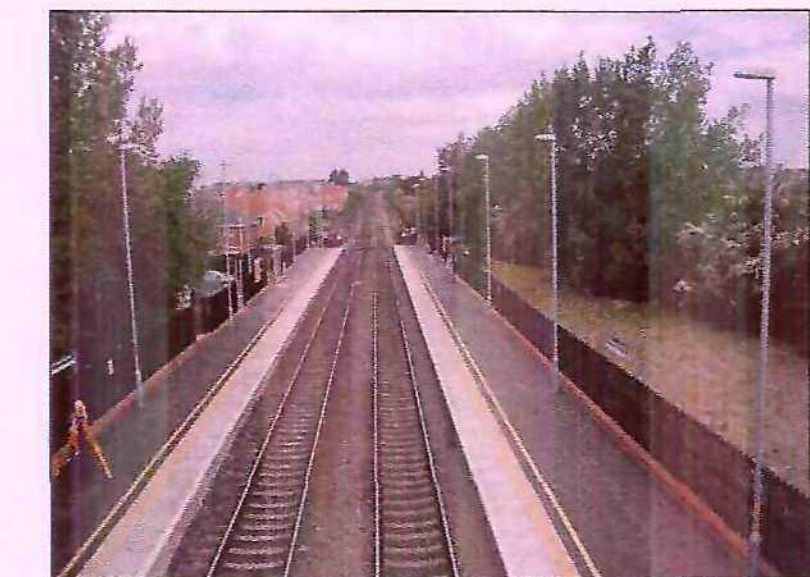
GENERAL VIEW FROM THE ROADBRIDGE LOOKING NORTH. EXISTING CROSSING IN THE BACKGROUND
