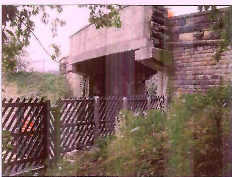
LOWFIELD ROAD OVERBRIDGE ABUTMENTS
