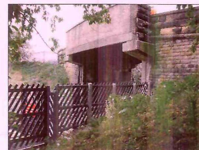
LOWFIELD ROAD OVERBRIDGE ABUTMENTS
