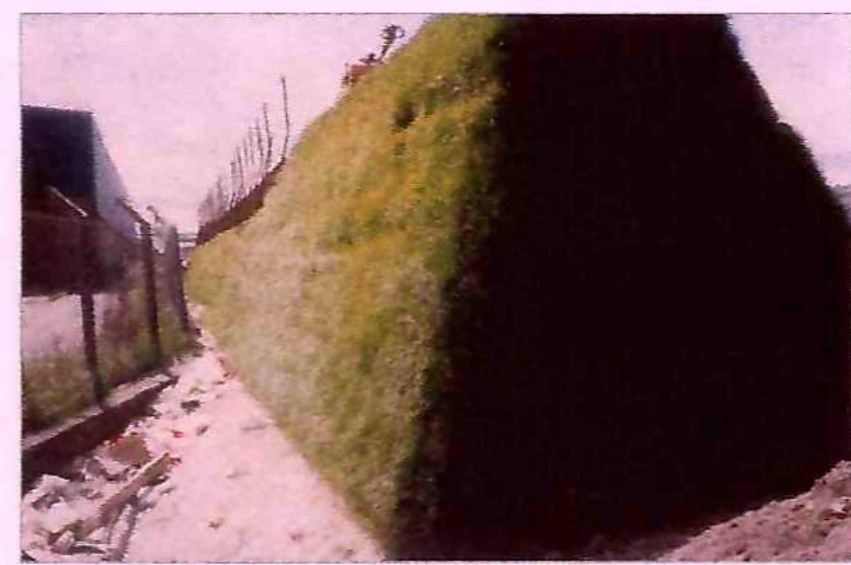
PHOTO OF TYPICAL REINFORCED EARTH STRUCTURE
