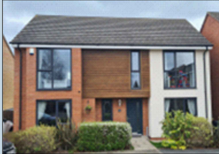
Photo Ref 01 Existing South West Facing, Front Elevation
