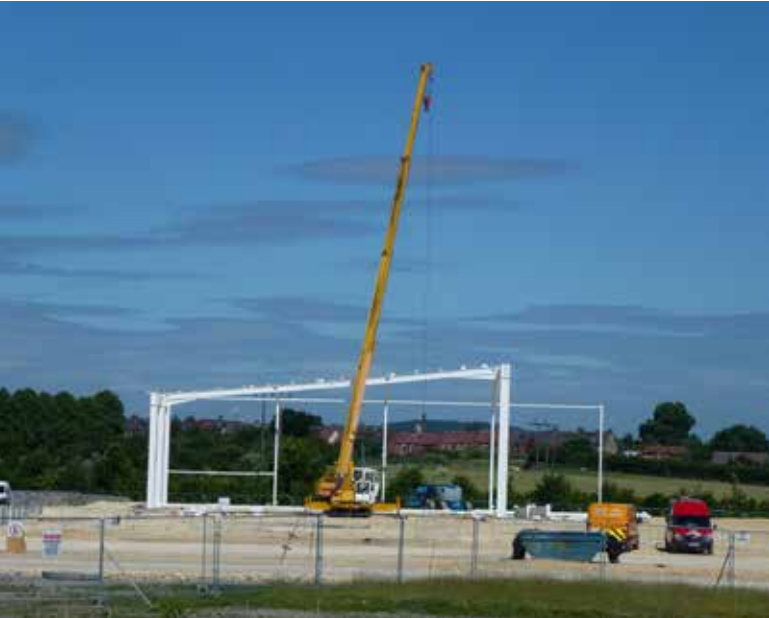
Below: Construction underway in wider development area
