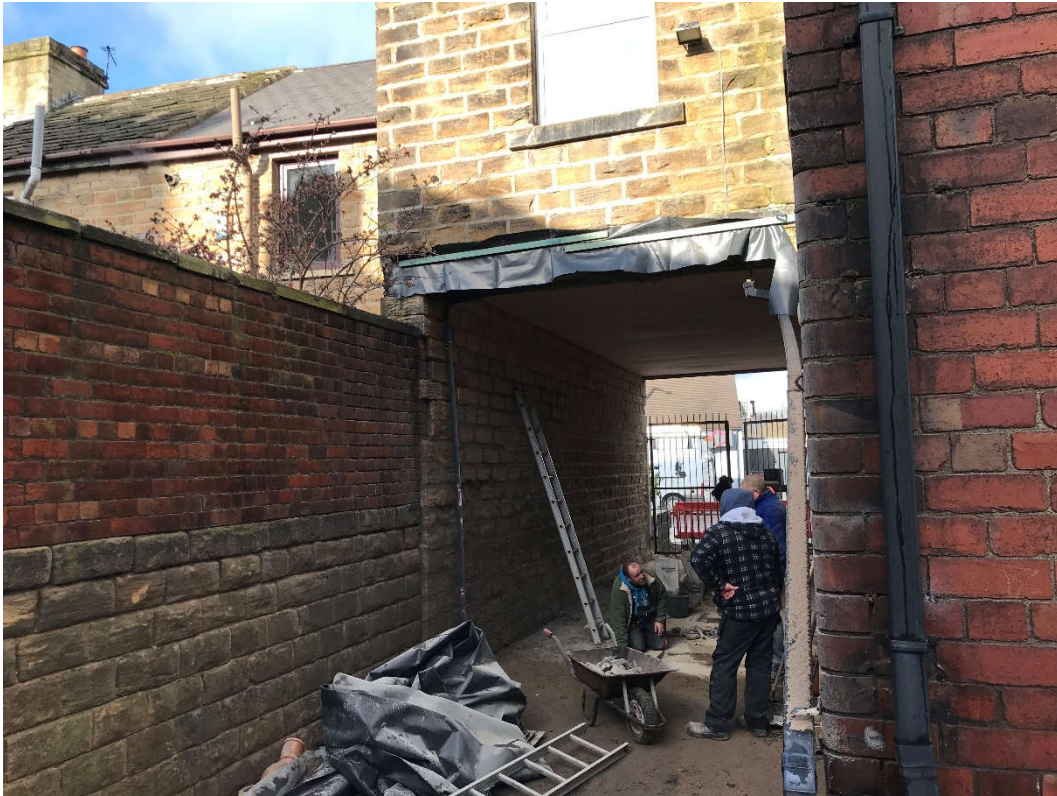
Fig 03. View of passageway from the rear.
