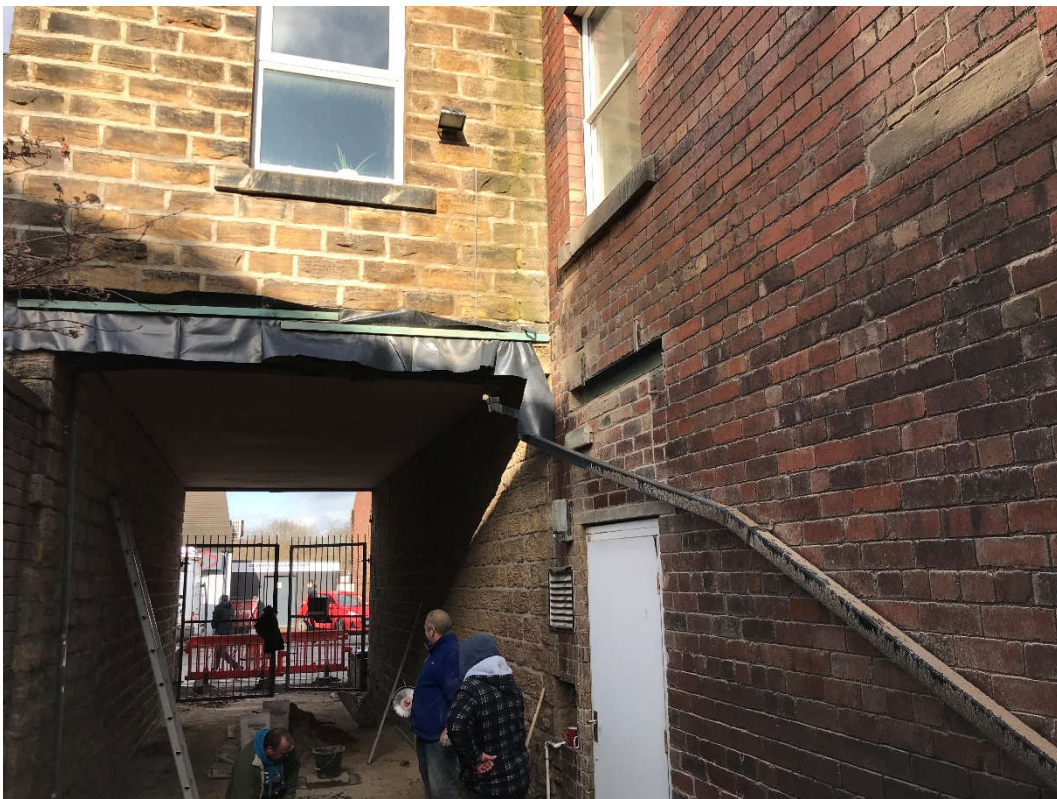
Fig 04. View of passageway from the rear.
