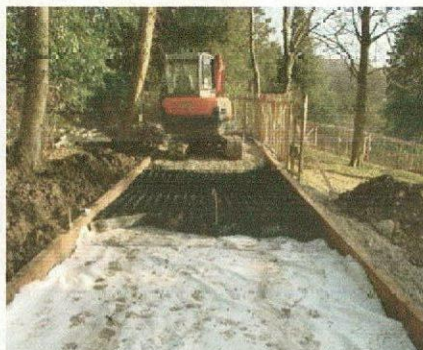
Fallbarrow Park, Windermere: CellWeb TRP® Installation
