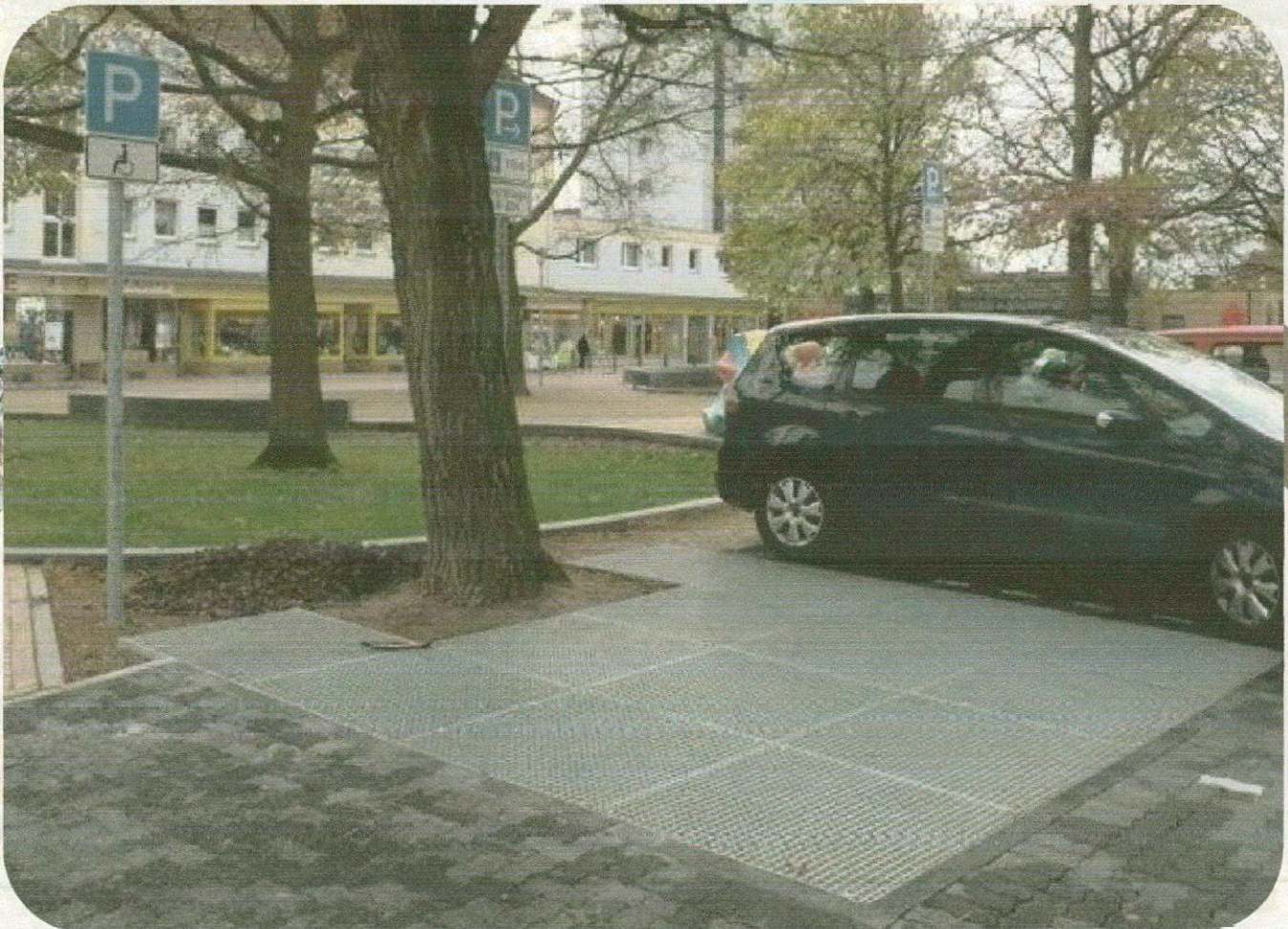
Light duty install in a carpark, heels-safe mesh finish.
