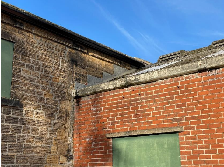
Photo 3 Flashing in good condition along western edge of B20b
