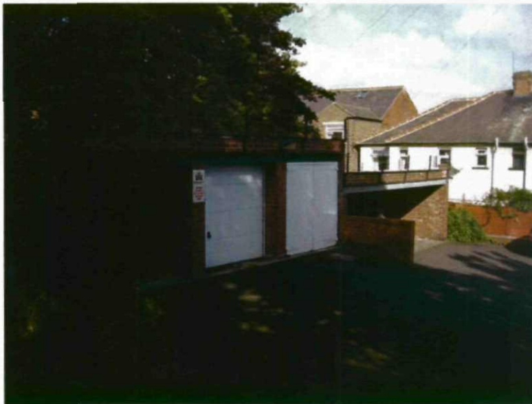
Photo 6: Buildings B3 (left) and B2 (right)
