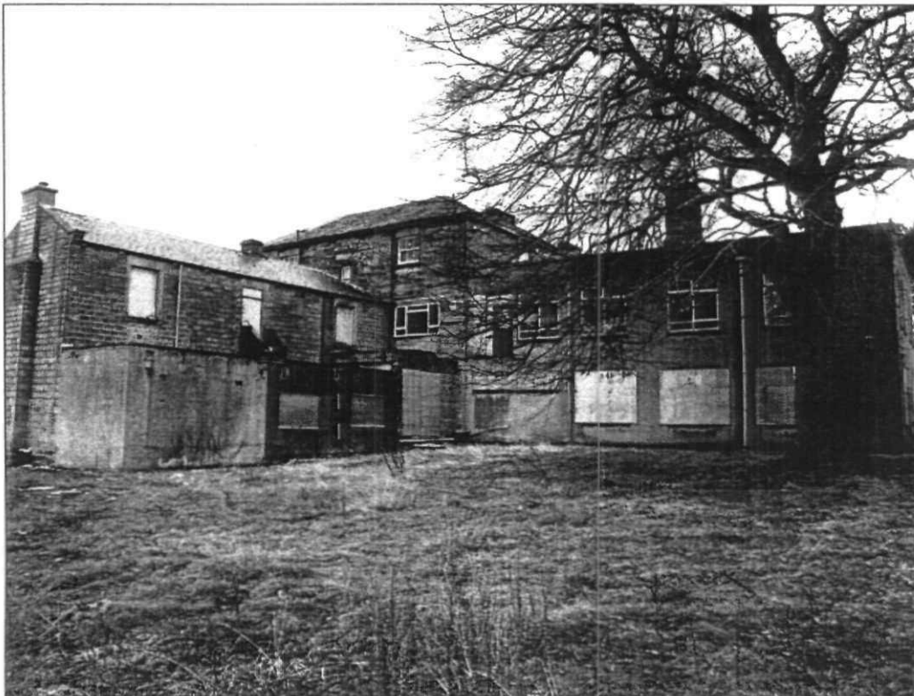
Fig. 26 Rear extension (on the right) and modern building (on the left)
