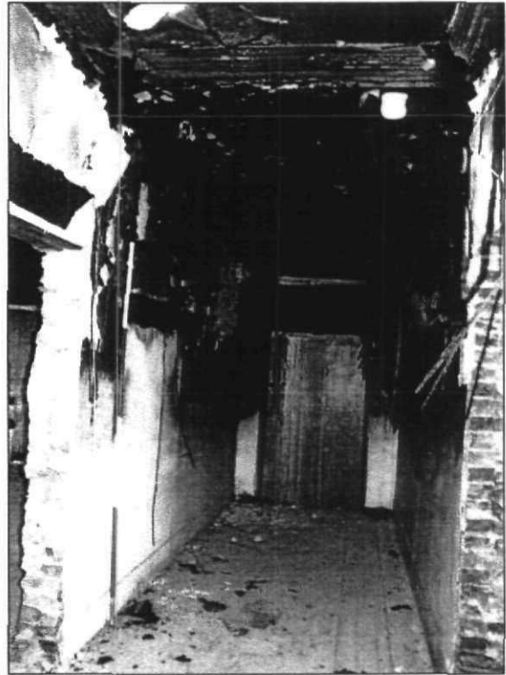
Fig. 35 Hallway on the first floor
