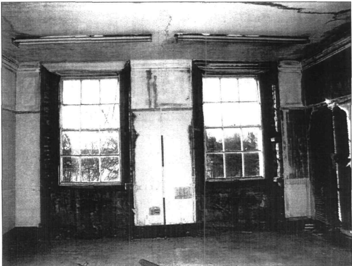
Fig.36 View of the south-western room on the first floor
