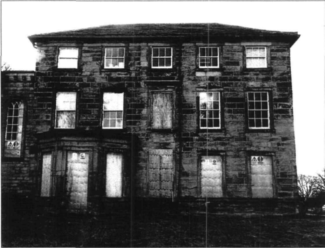
Fig. 27 Western elevation of Brierley Hall
