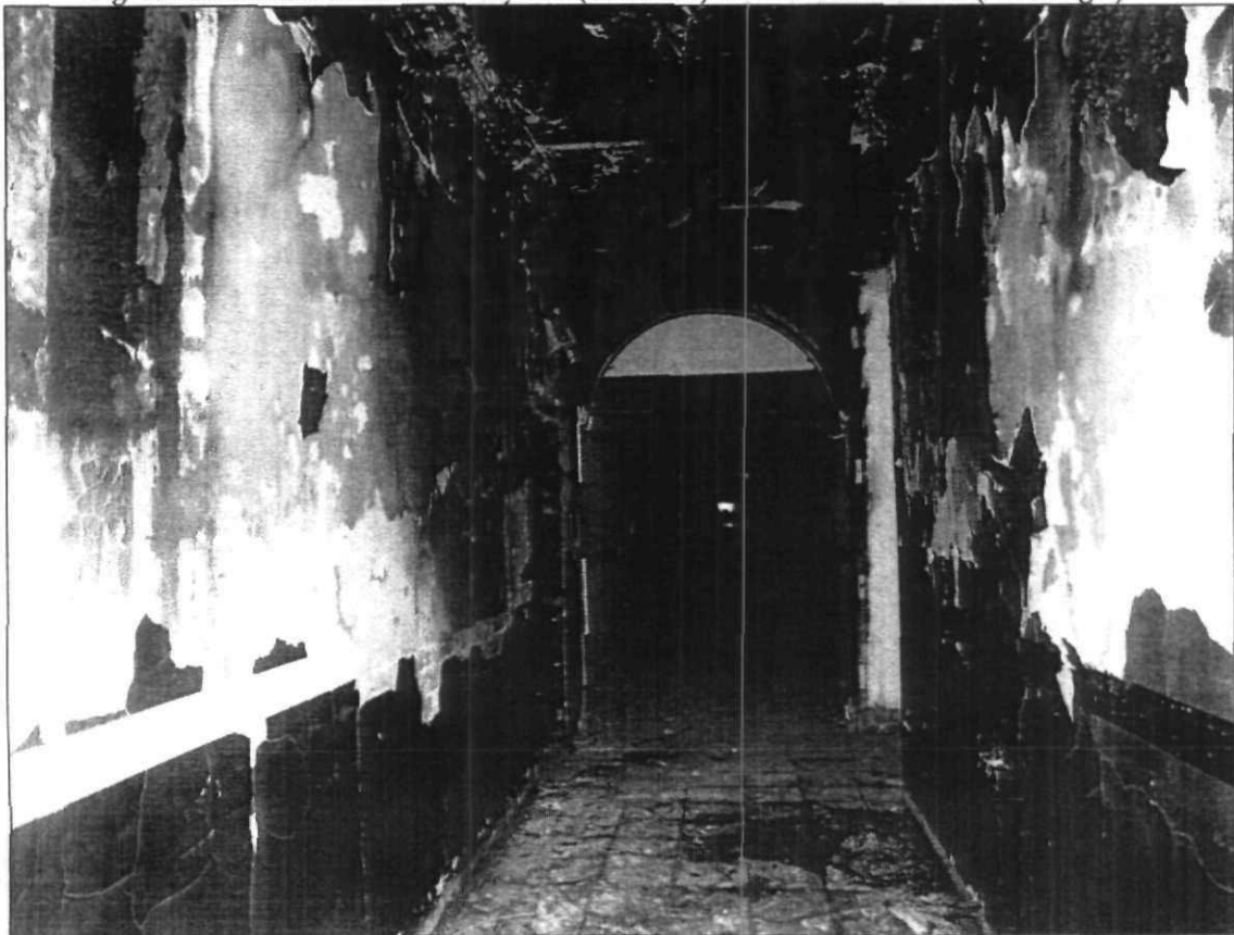
Fig. 29 Hallway on the ground floor
