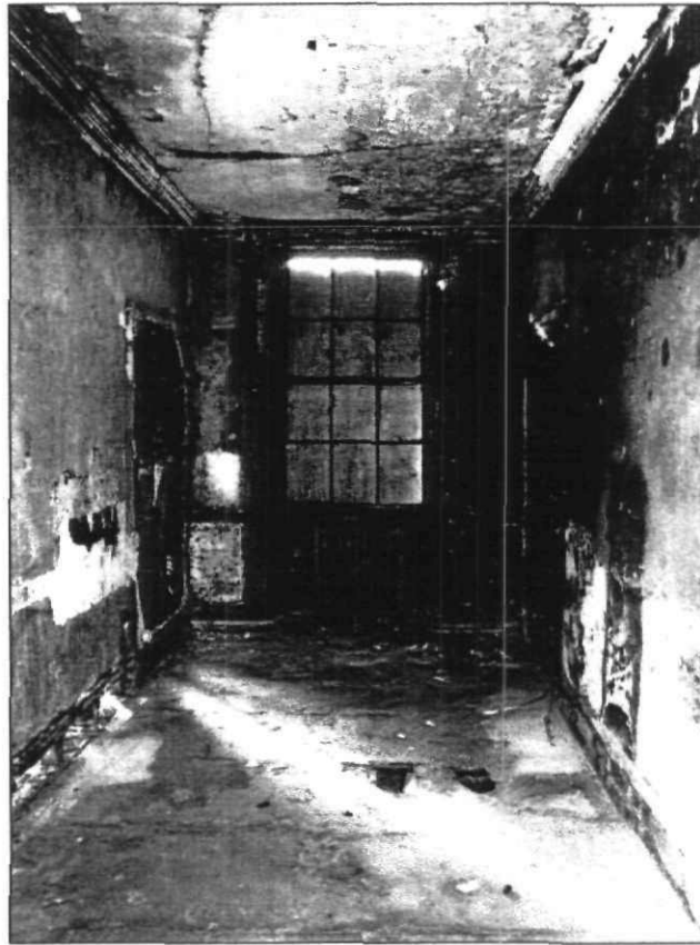
Fig.37 Window on the central bay of the first floor with additional radiator
