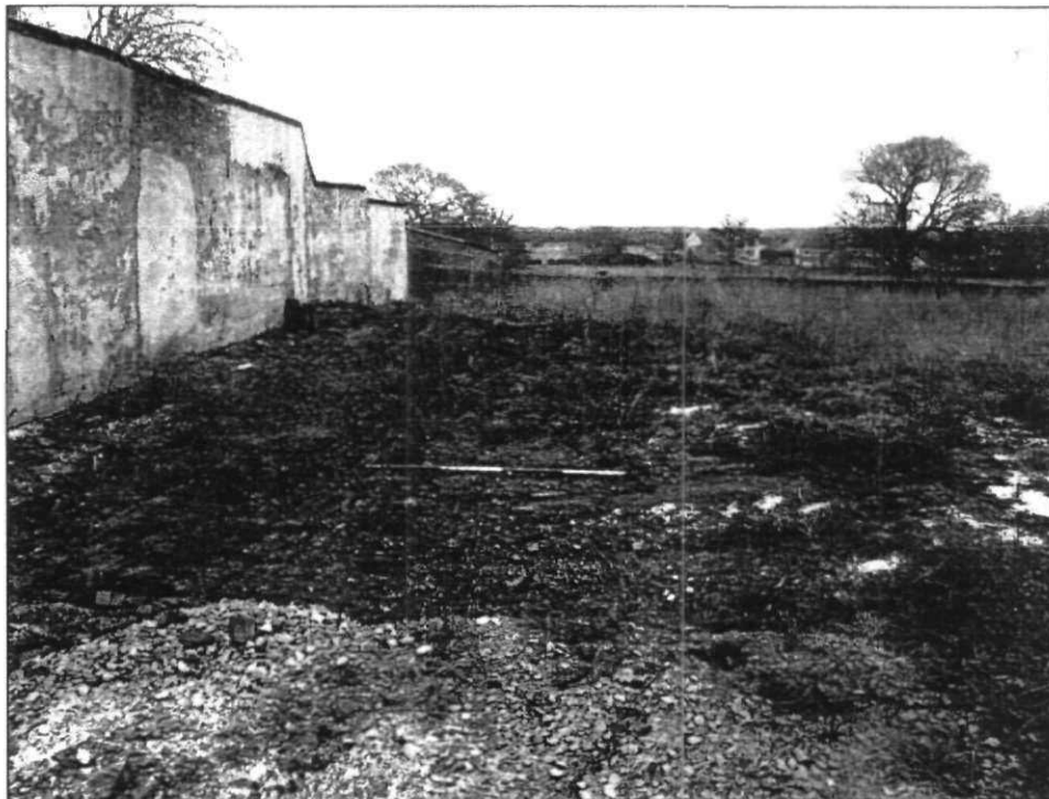
Fig. 22 Area of the demolished building along the North boundary of the site that is marked on OS maps from 1893. Also shows the brick wall that may be part of the original garden boundary.
