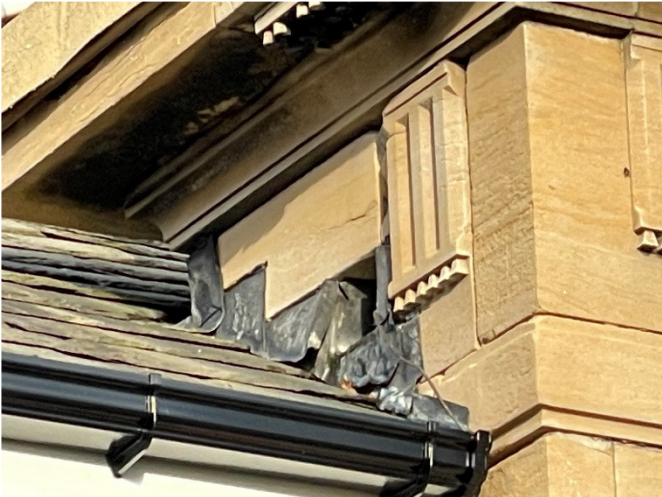
Figure 9 Showing raised flashing around the sandstone entrance
