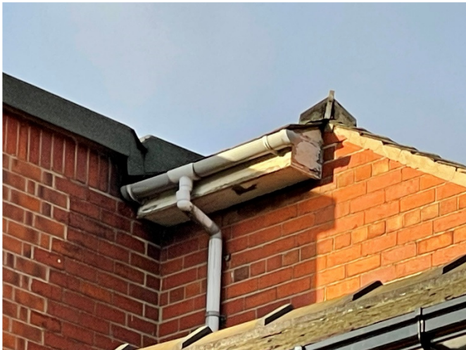
Figure 6 Showing small section of worn fittings with gaps between them and the wall
