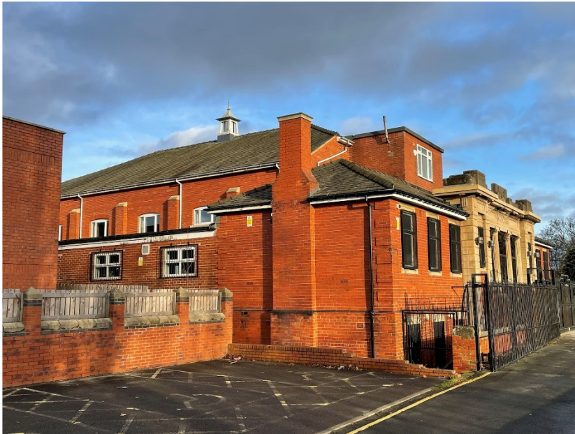
Figure 3 General view of the building on site.
