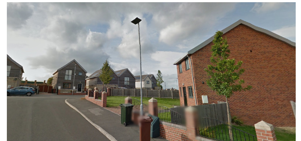
New mottled red brick and cedar clad units in first phases of SYHA regeneration development
