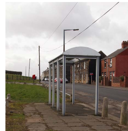
Exposed bus stop on site
