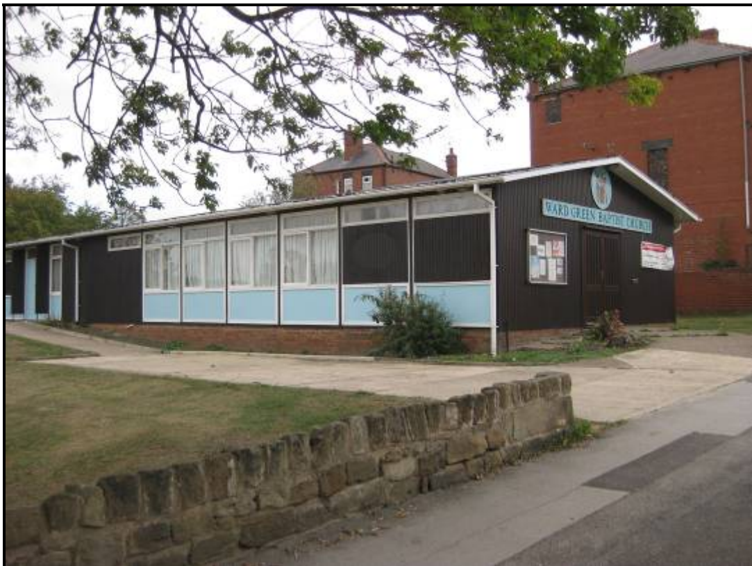
Figure 14 - Ward Green Baptist Church to the east of the site
