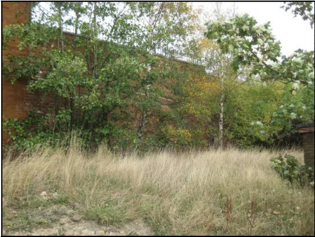
Figure 4 - Southern boundary showing high retaining wall
