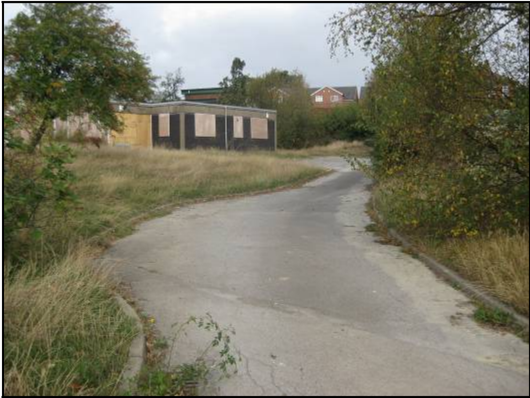
Figure 2 - Existing entrance to the school
