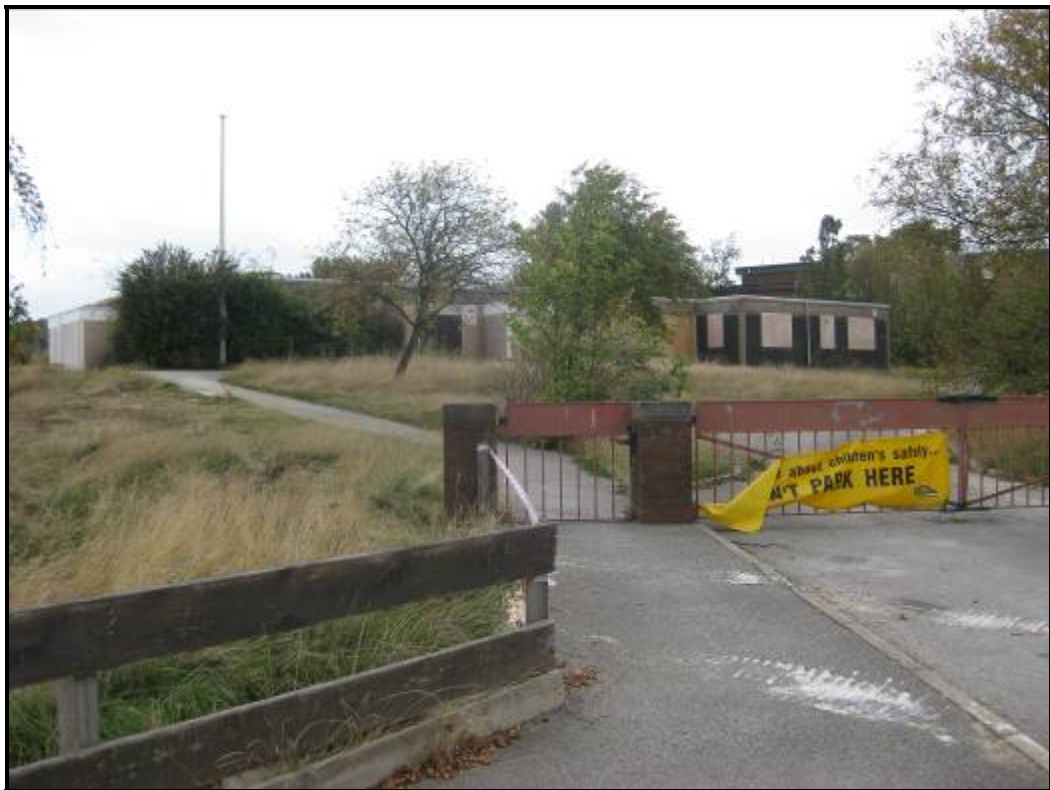
Figure 7 - Eastern elevation and former entrance to the school.
