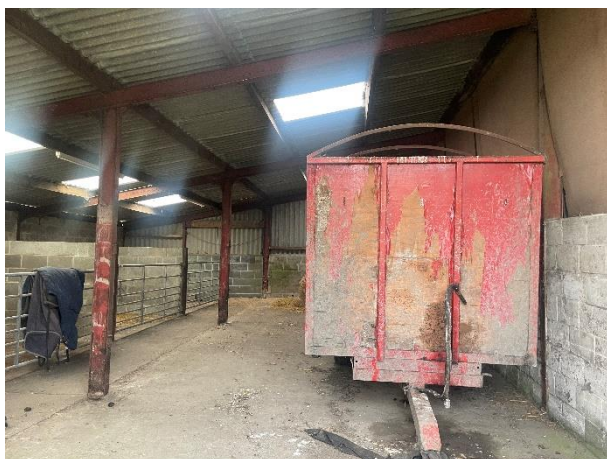
Photo 7: Interior of the building.
