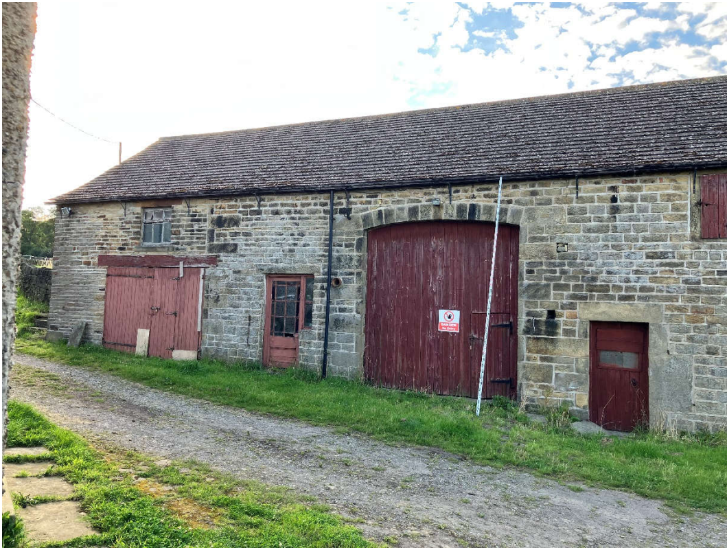
Fig 09. Barn – South Elevation (west end).
