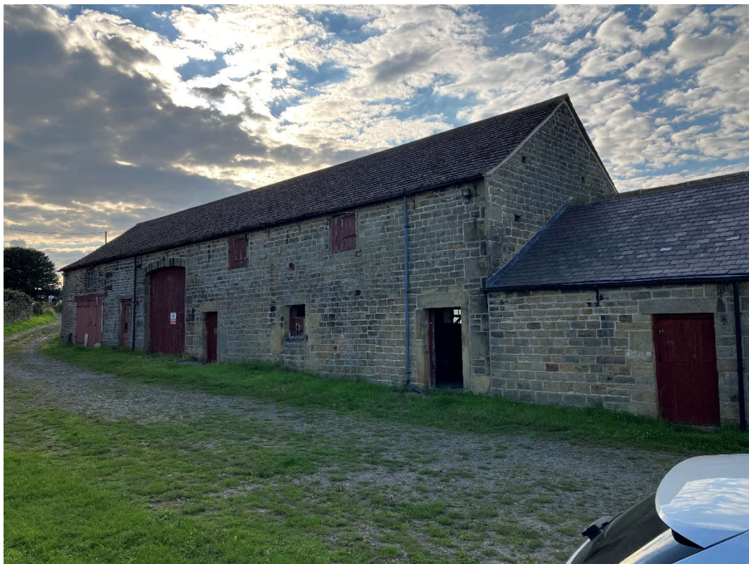
Fig 10. Barn – South Elevation.
