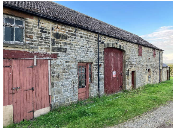
Main Barn south elevation
