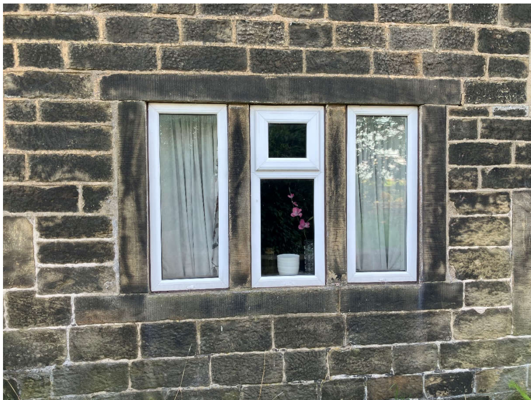
Fig 04. Farmhouse – Typical view of existing Upvc window frames.
