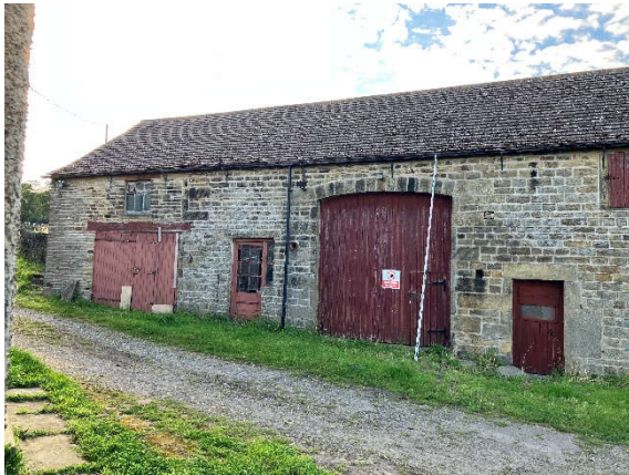
Main Barn south elevation
