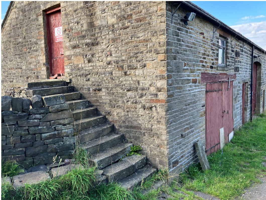
Fig 07. Barn – West gable and stone steps.
