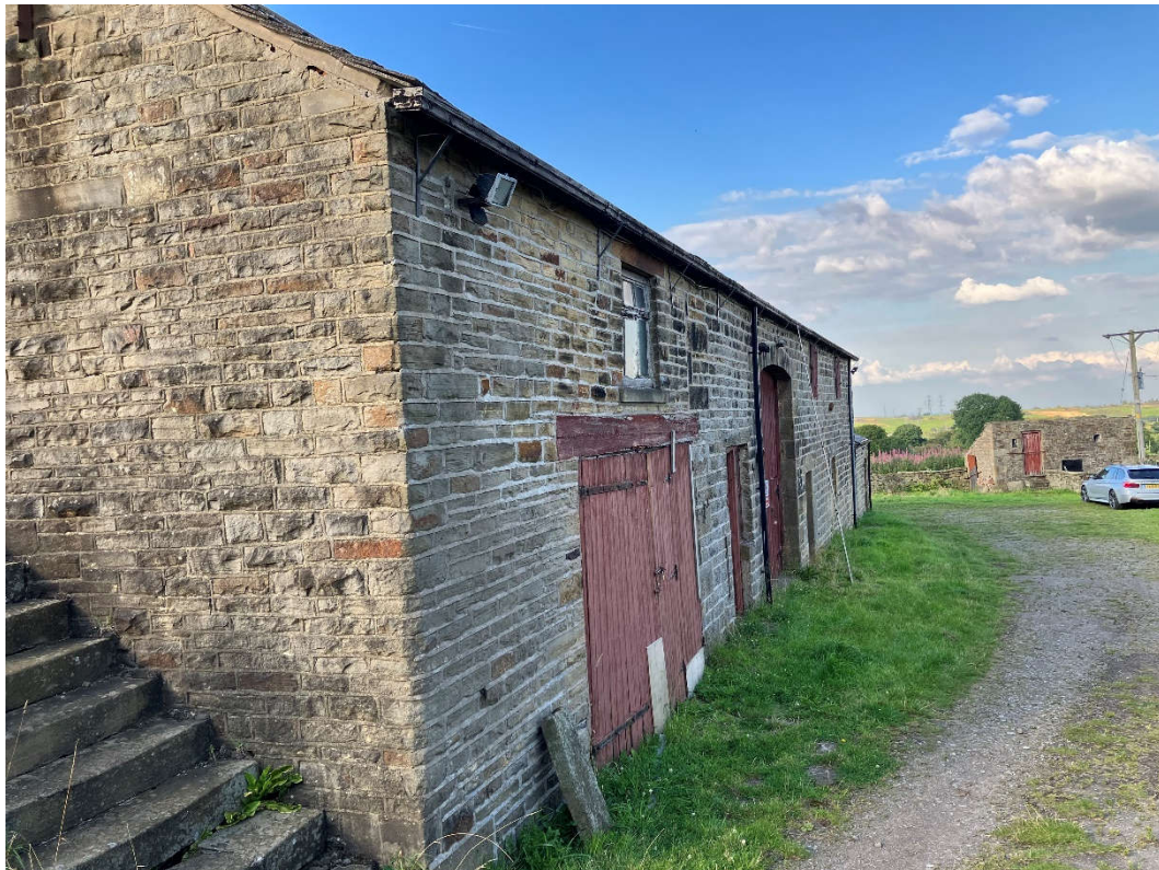
Fig 08. Barn – South Elevation.
