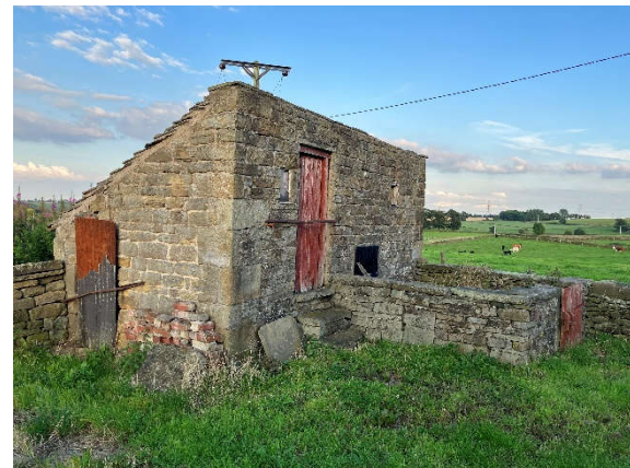
Small outbuilding to east.
