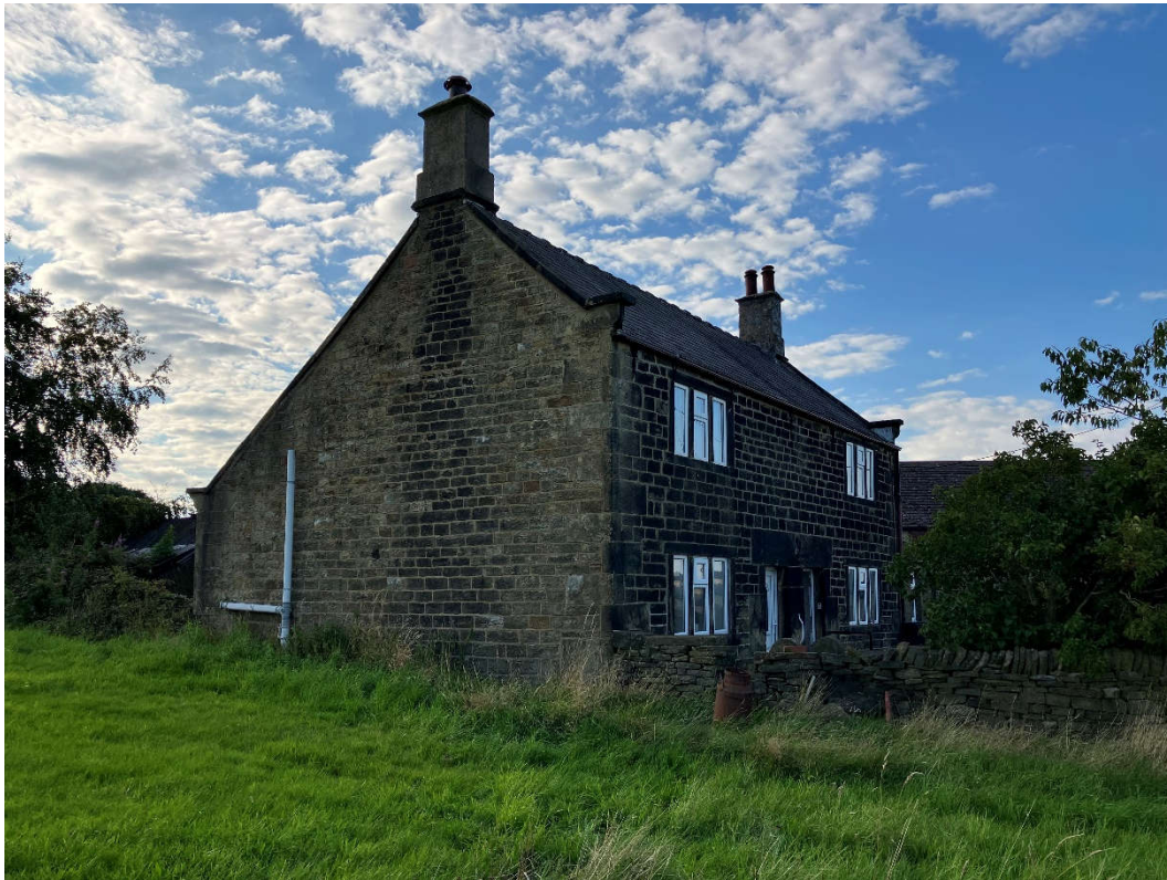
Fig 01. Farmhouse – Gable South, and East Elevation.
