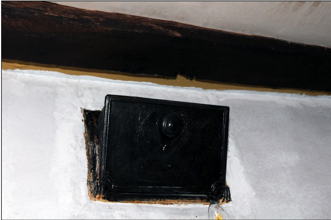
Plate 6: Detail of Victorian cast iron vent (Image 011).
