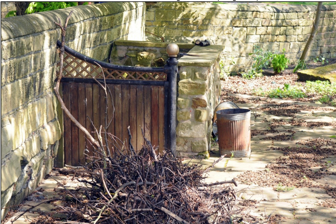
Plate 5: Detail of relocated stable partition (Image 109).
