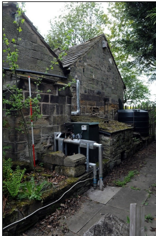
Plate 11: General view of the north elevation of Unit 3 and Unit 2 (Image 124)
