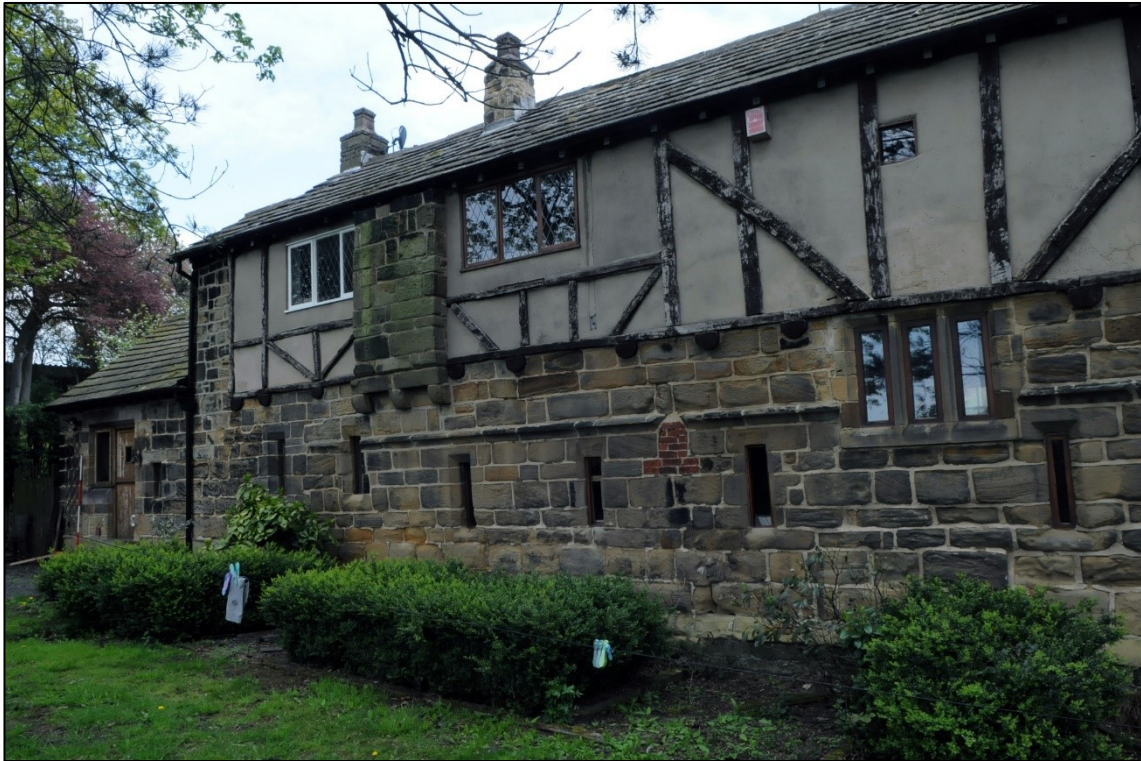
Plate 4: General view of northern end of west facing elevation (Image 062).
