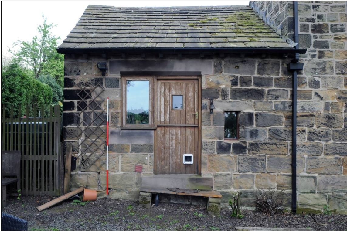
Plate 10: Detail of northern end of western elevation (Image 047)
