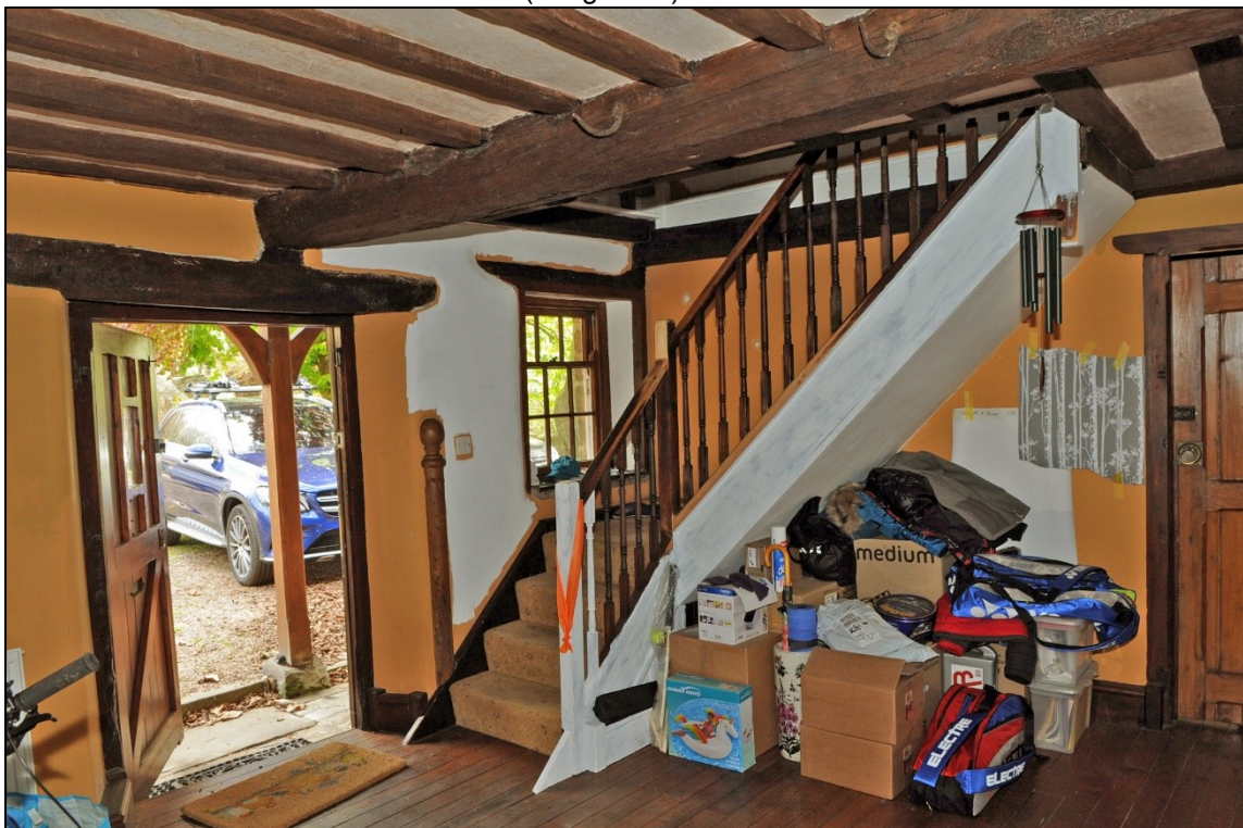
Plate 7: General view of the interior of the coach house, note the hooks in the ceiling beams. (Image 013).
