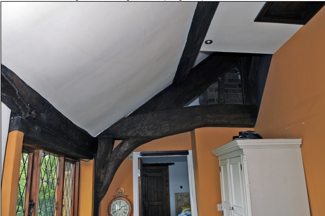
Plate 9: Detail of roof truss (Image 022).
