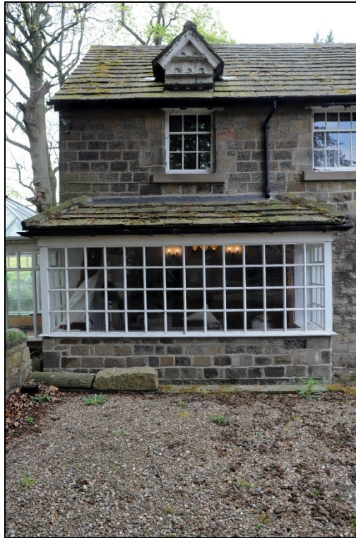
Plate 3: General view of the southern end of the eastern elevation (Image 110).
