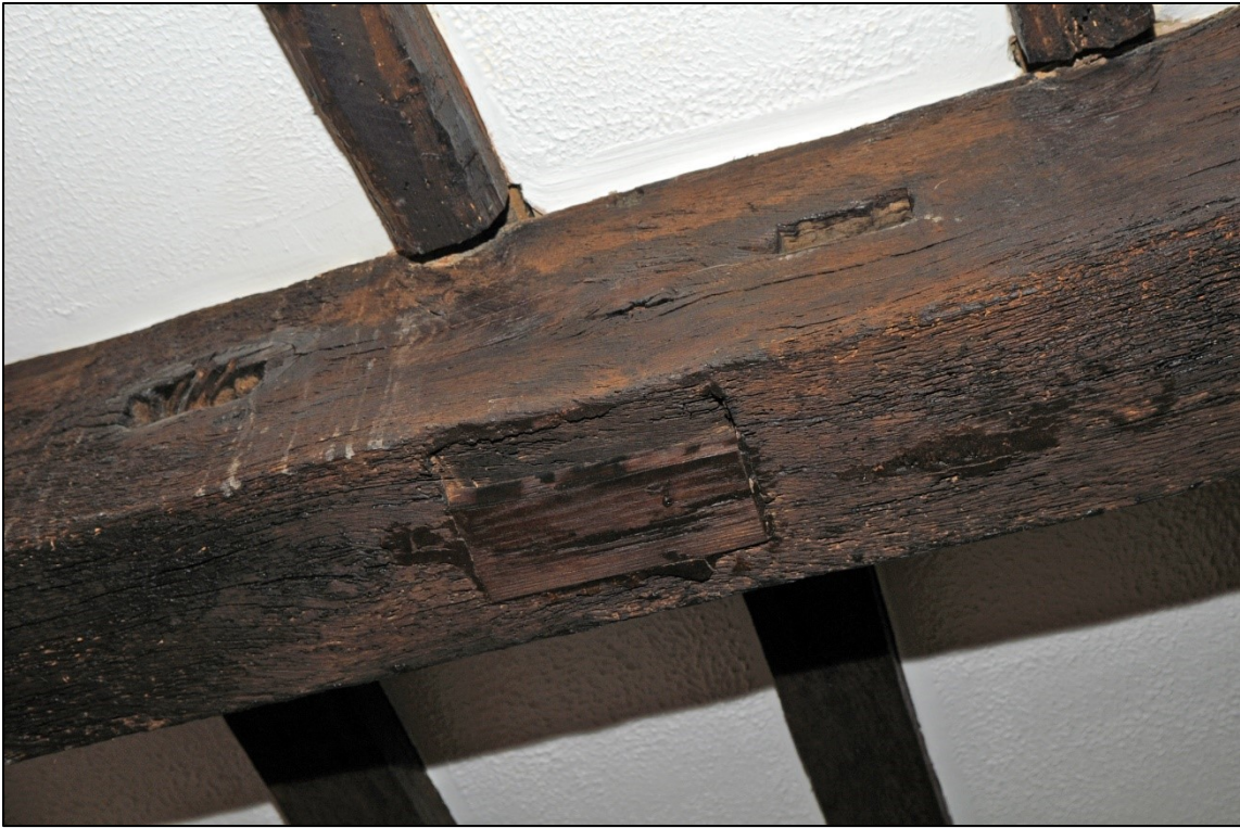
Plate 8: Detail of ceiling beam showing mortices (Image 021).
