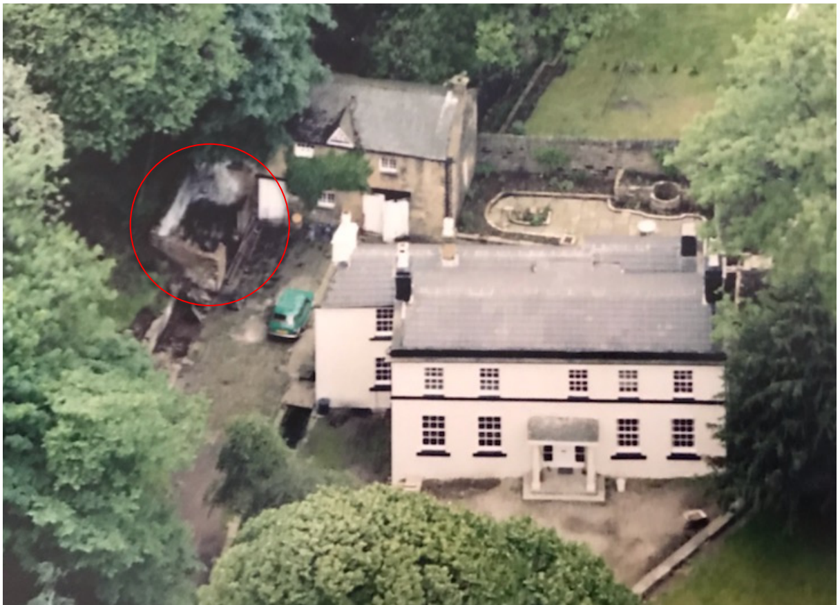
Red circle shows part of building which no longer exists
