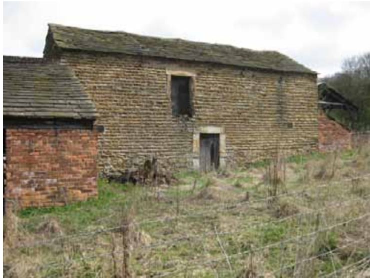
Photograph 68: Shows the South-west Elevation of Agricultural Building 'B'. The main building consists of coursed sandstone masonry with timber floor and trusses, supporting a slate roof. Several brickwork extensions have been added on to the main building to each elevation.
