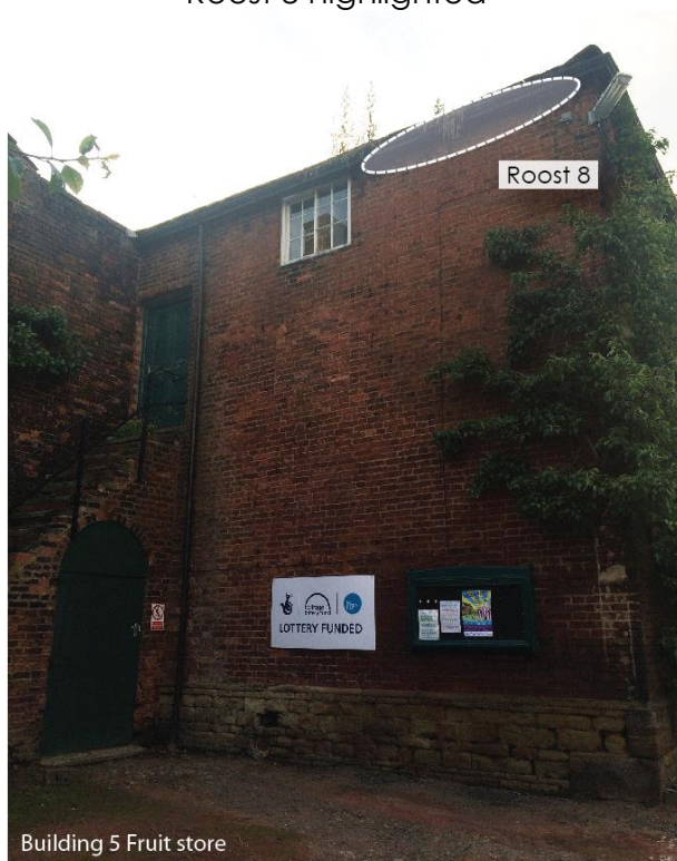
Figure 6 Southern elevation of Building 5 – Roost 8 highlighted
