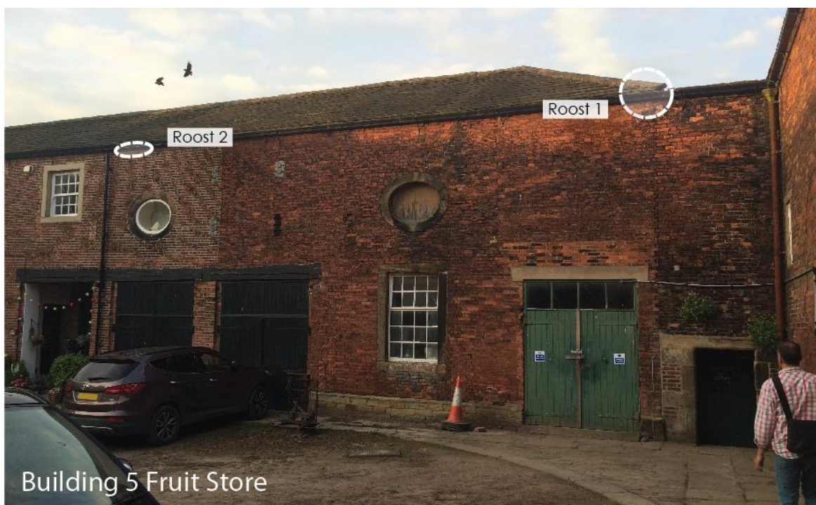
Figure 3 Western elevation of Building 5 - Roosts 1 & 2 highlighted
