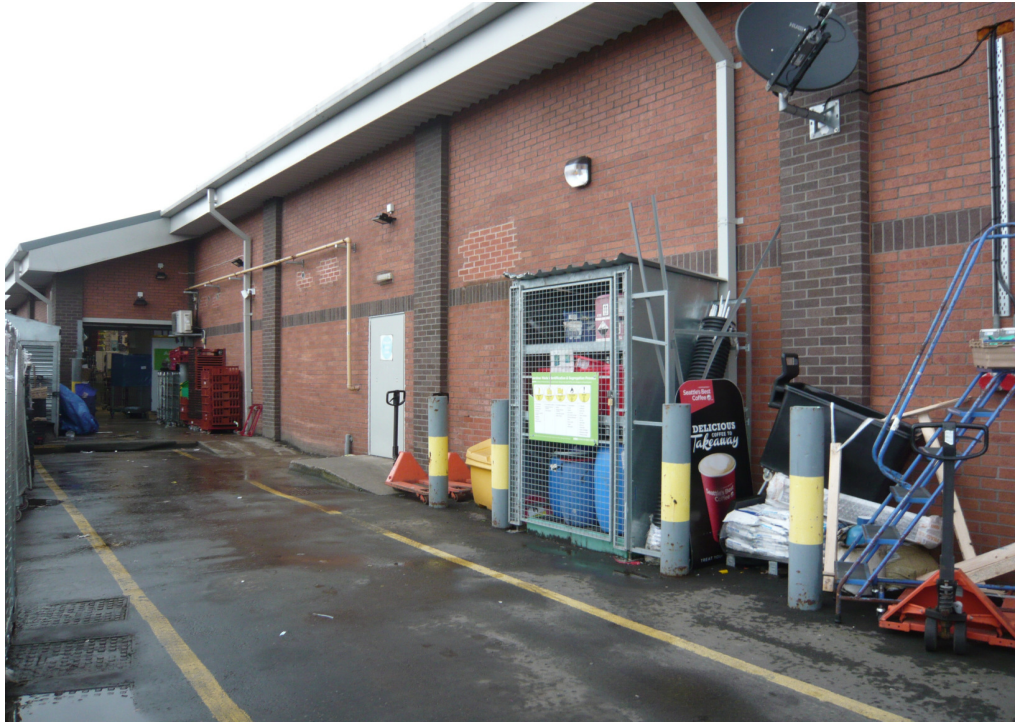
View of the existing service/marshalling area
