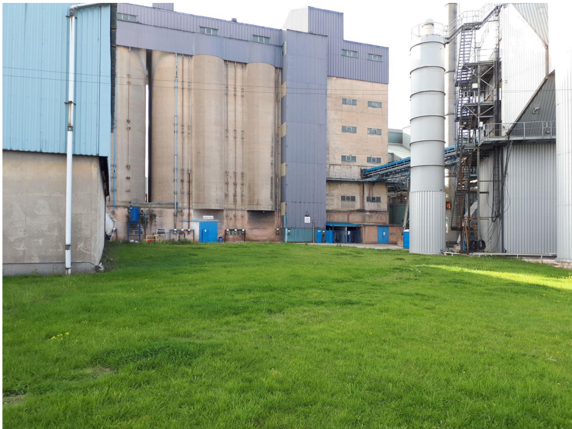
Photograph 1 Site Location for Plant Room: from grassy area looking south towards existing batch plant, with sand store on the left and filter unit on the right
