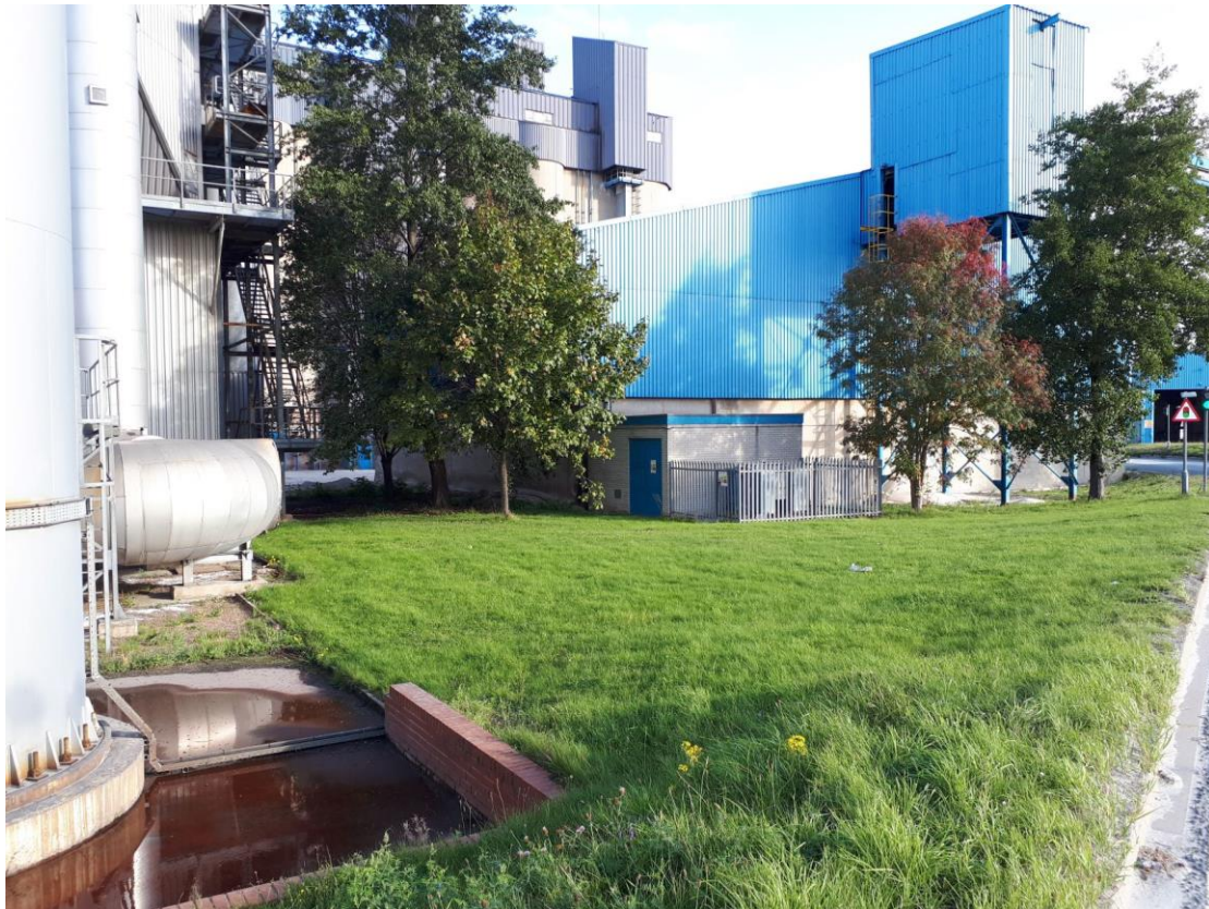
Photograph 3 Site Location for most southerly Heat Exchanger: from the edge of the site road looking north
