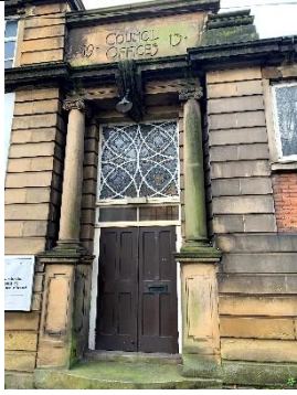
Figure 17 – Unused entrance between Town Hall and Paramount
