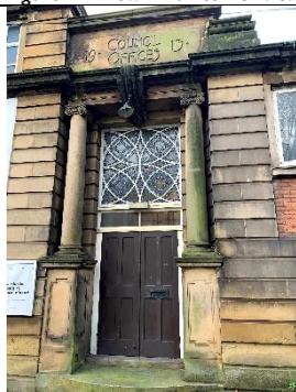
Figure 4 – Unused entrance between Town Hall and Paramount
