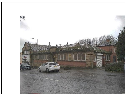
Figure 15 – Town Hall from Shrewsbury Road
