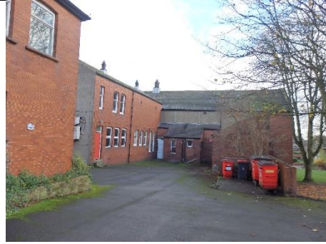
Figure 18 – Rear external view of service courtyard
