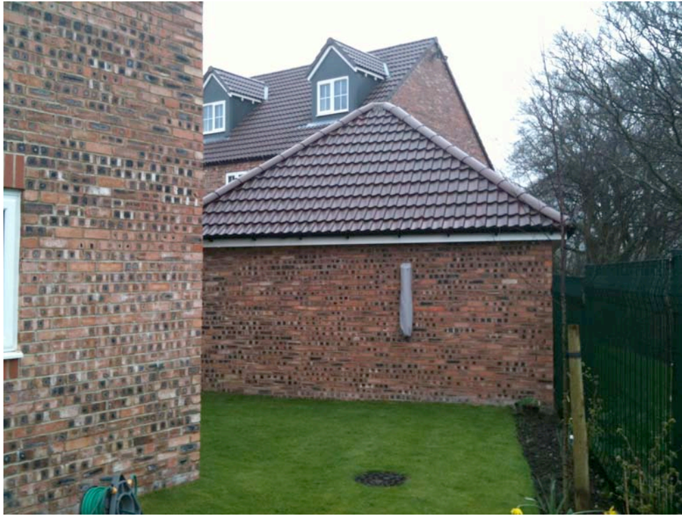
Part rear view showing adjacent garage
