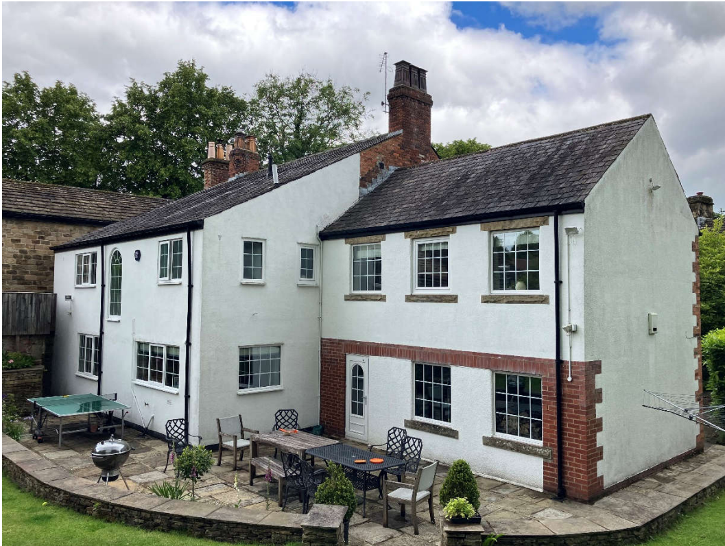
01. View of rear of house looking north west.
