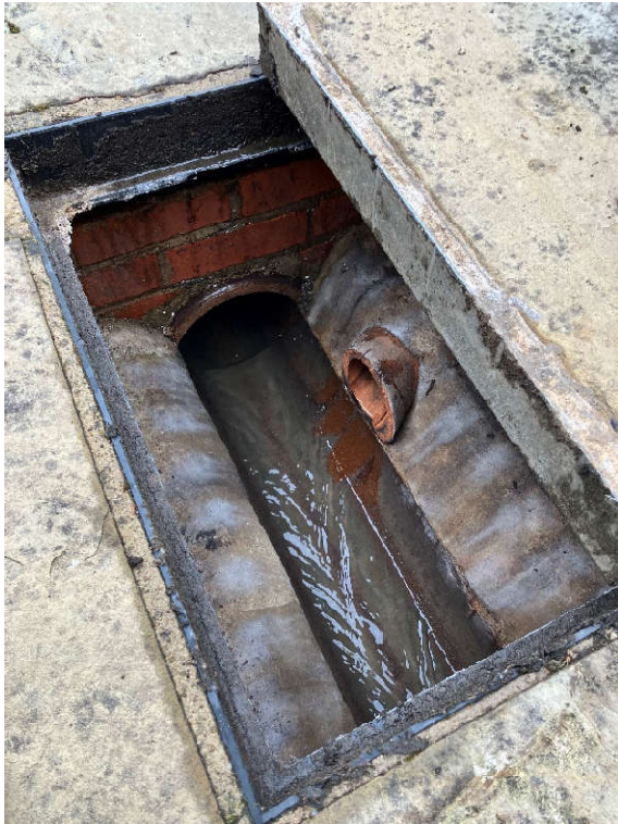
03. MH01 looking south.
