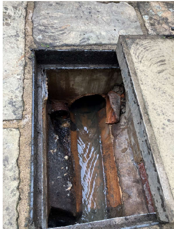
06. MH02 looking south.
