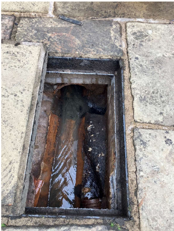
05. MH02 looking north.
