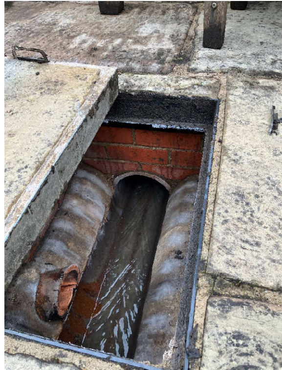
04. MH01 looking north.
