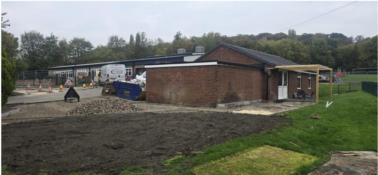
Photograph 3: General view of site
