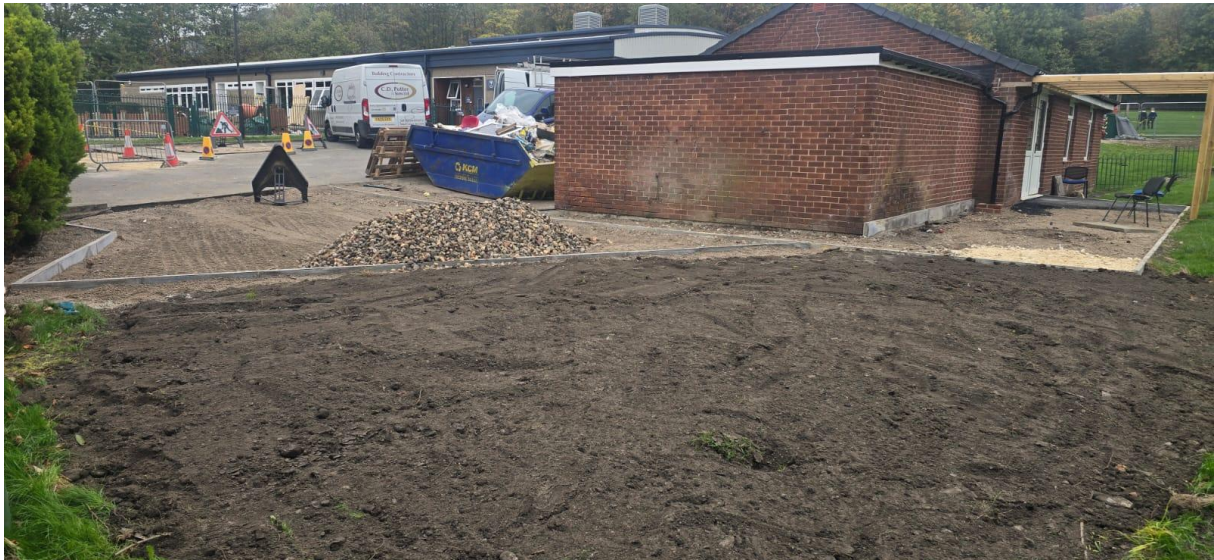
Photograph 2: General view of site
