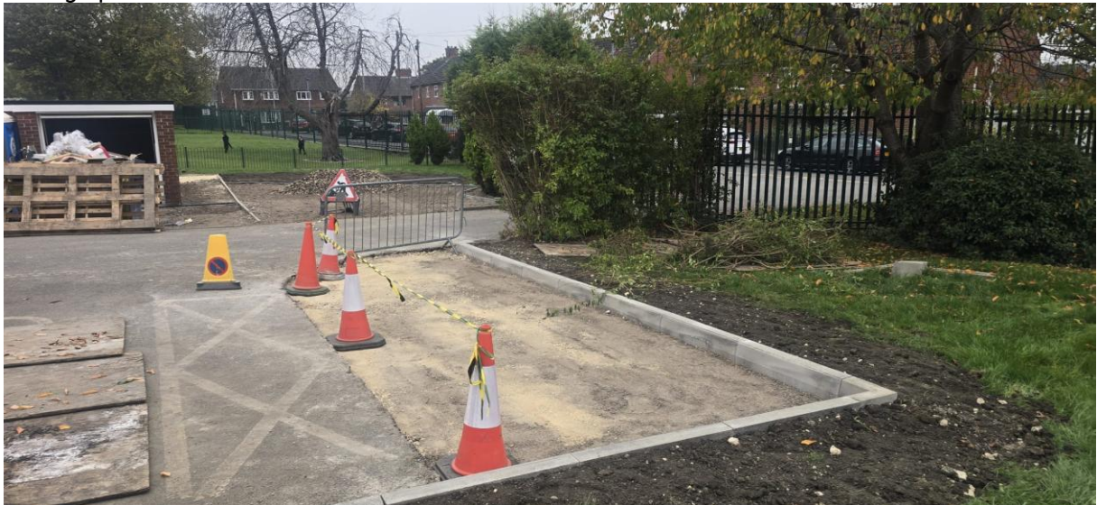
Photograph 4: General view of site
