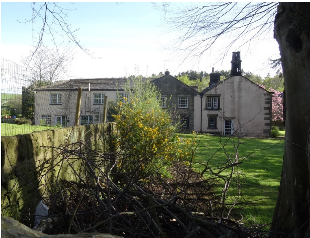
Figure 3.1 Nether Mill House and Later Rear Annex on left hand side (proposed for demolition)
