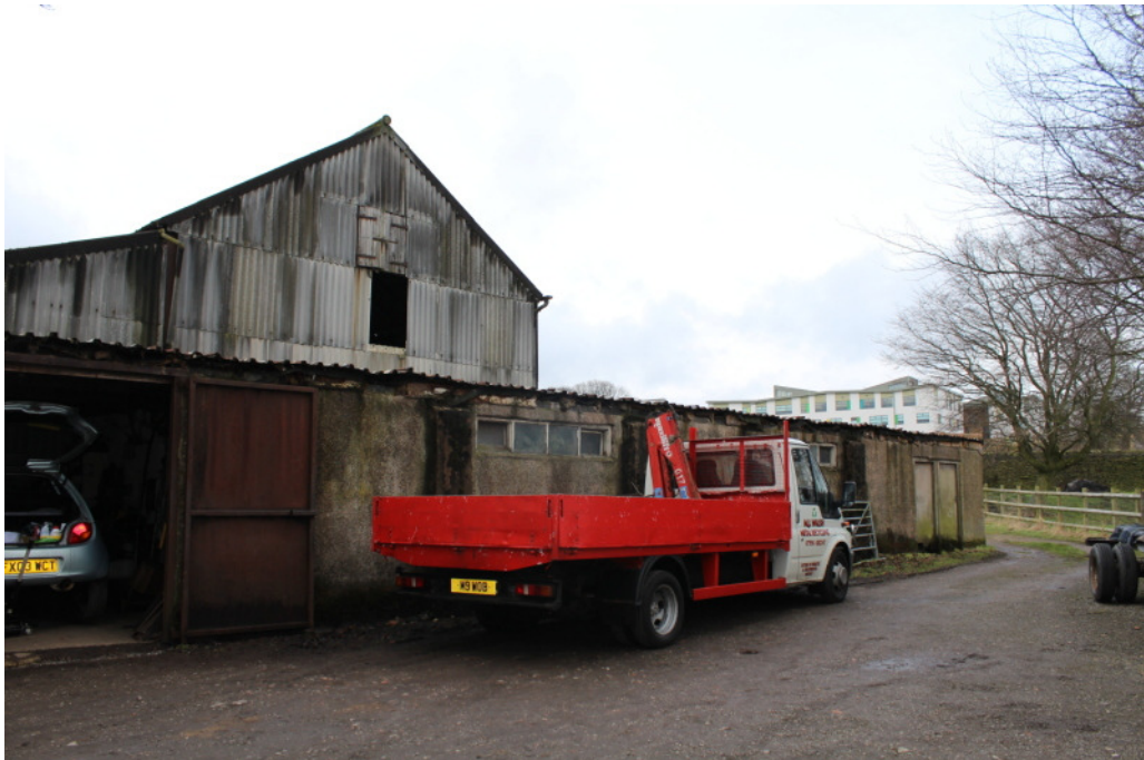
Figure 3.4 Nether Mill House - Adjacent Agricultural Buildings
