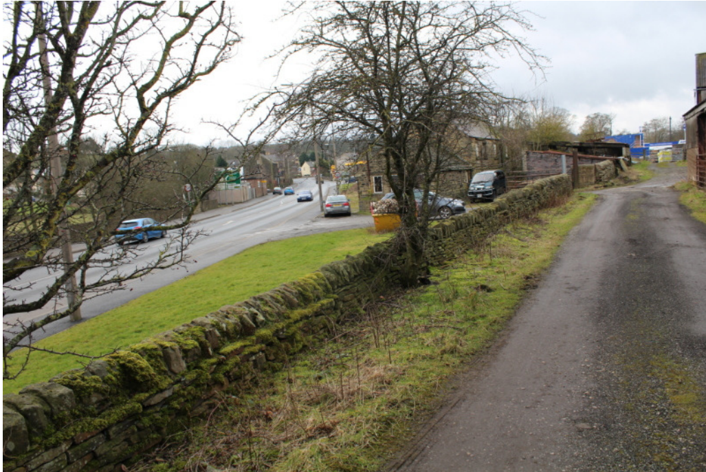
Figure 3.3 Existing Dry Stone Wall to the South-West of Nether Mill House
