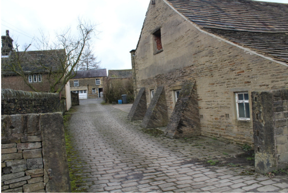
Figure 3.6 Nether Mill Barn
