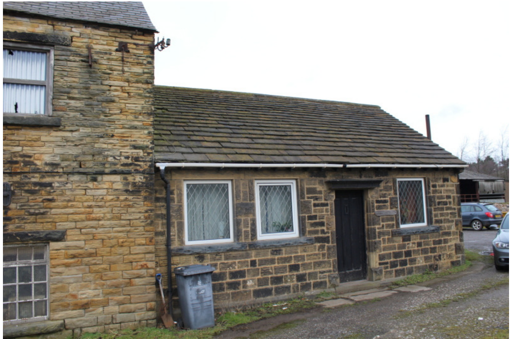
Figure 3.9 Adjacent Single Storey Cottage
