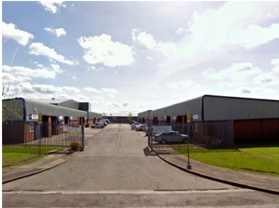
Goldthorpe Industrial Estate
