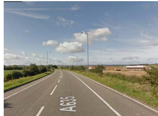
View looking down Dearne Valley Parkway A635 towards Hollygrove Roundabout
