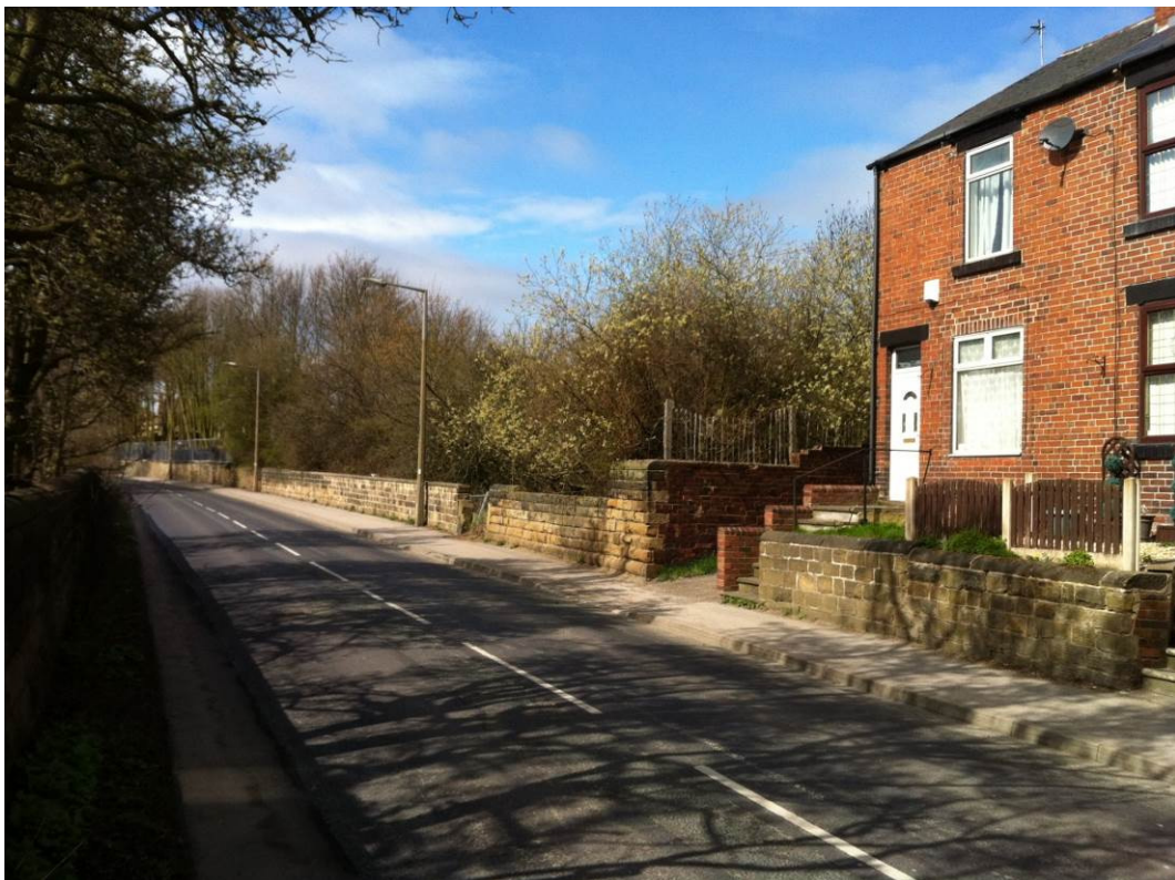
02. Site frontage to Common Road looking west with Royd View Cottages in foreground.
