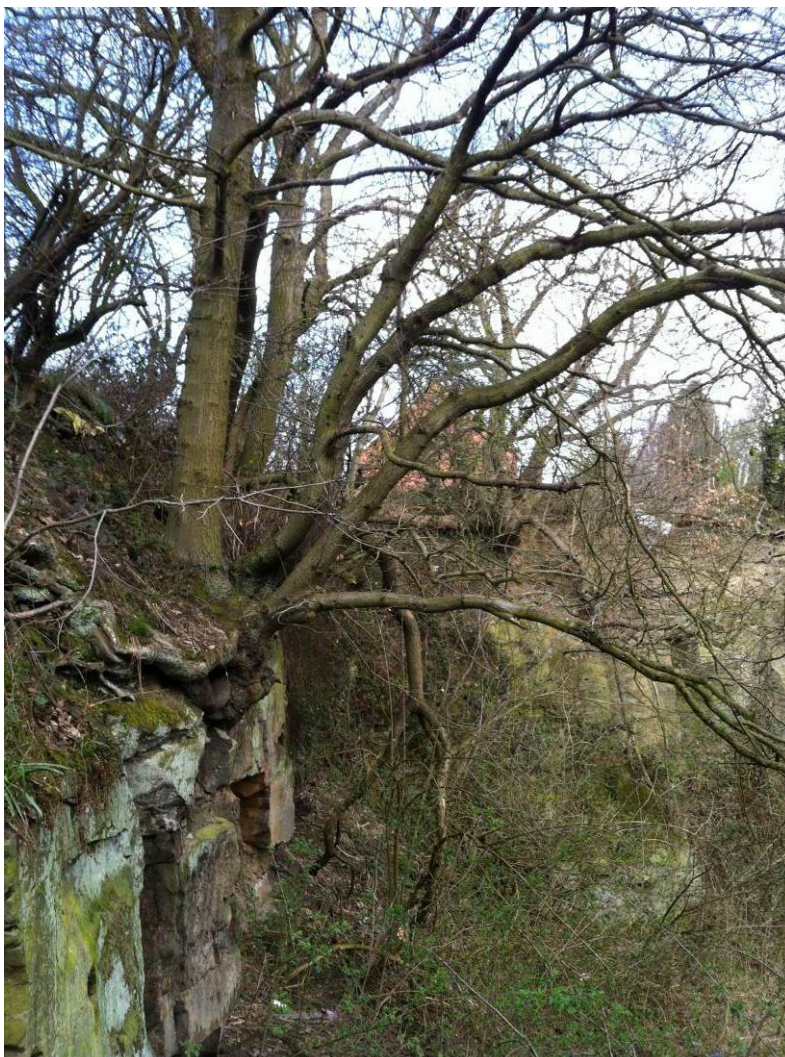
08. View of T38 showing overhanging branches to be removed.
