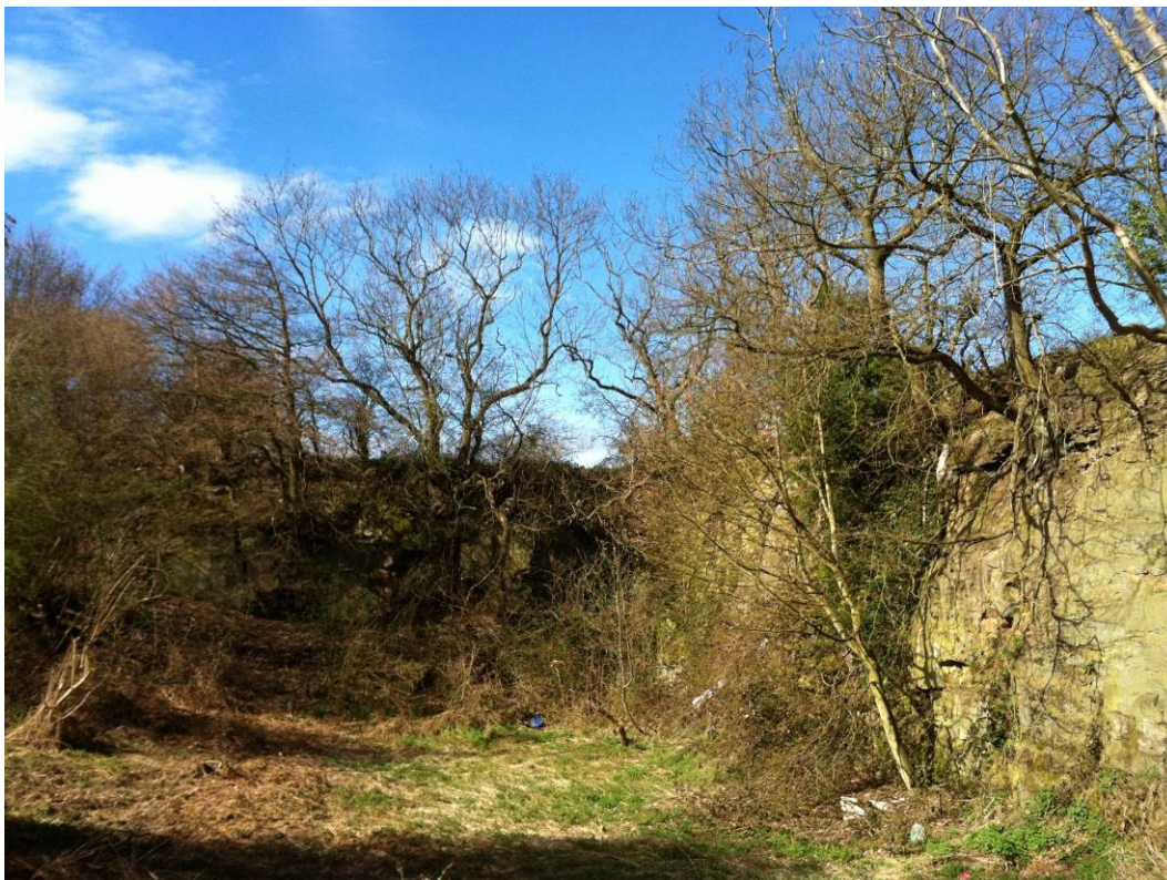
07. View of quarry floor to rear looking south west and showing rear quarry wall and typical arrangement of trees.
