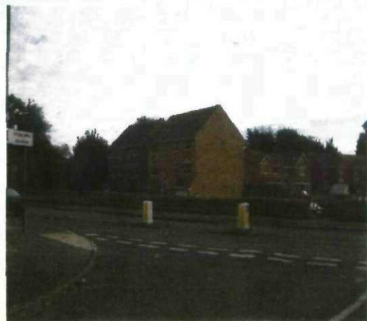
Fig 8 Recent development to the south of Barnsley Road
