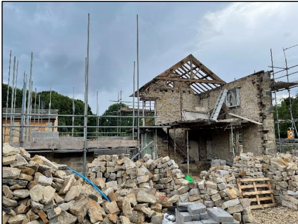
Figure 3: The building viewed from the east.
