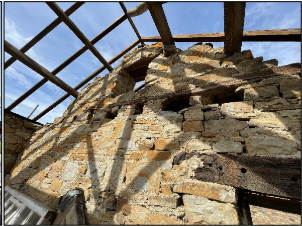
Figure 7: The joist holes in the walls.
