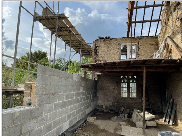
Figure 4: The new build walls to the southeast of the building.
