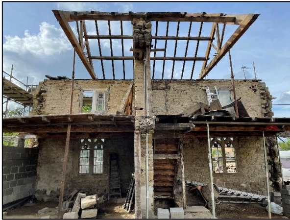
Figure 6: The partially demolished walls of the building.
