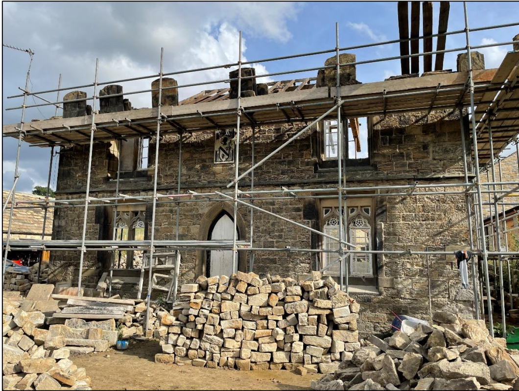
Figure 2: The remaining northwest elevation of the building.
