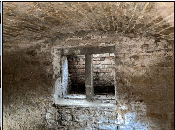
Figure 9: The stonework and missing window within the cellar.
