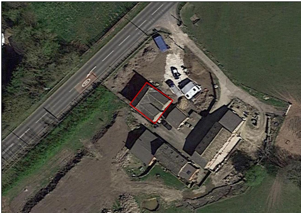
Figure 1: Showing the building covered by this survey (old image from before works began).
