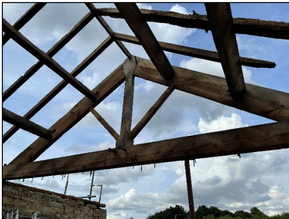
Figure 8: The exposed roof timbers.
