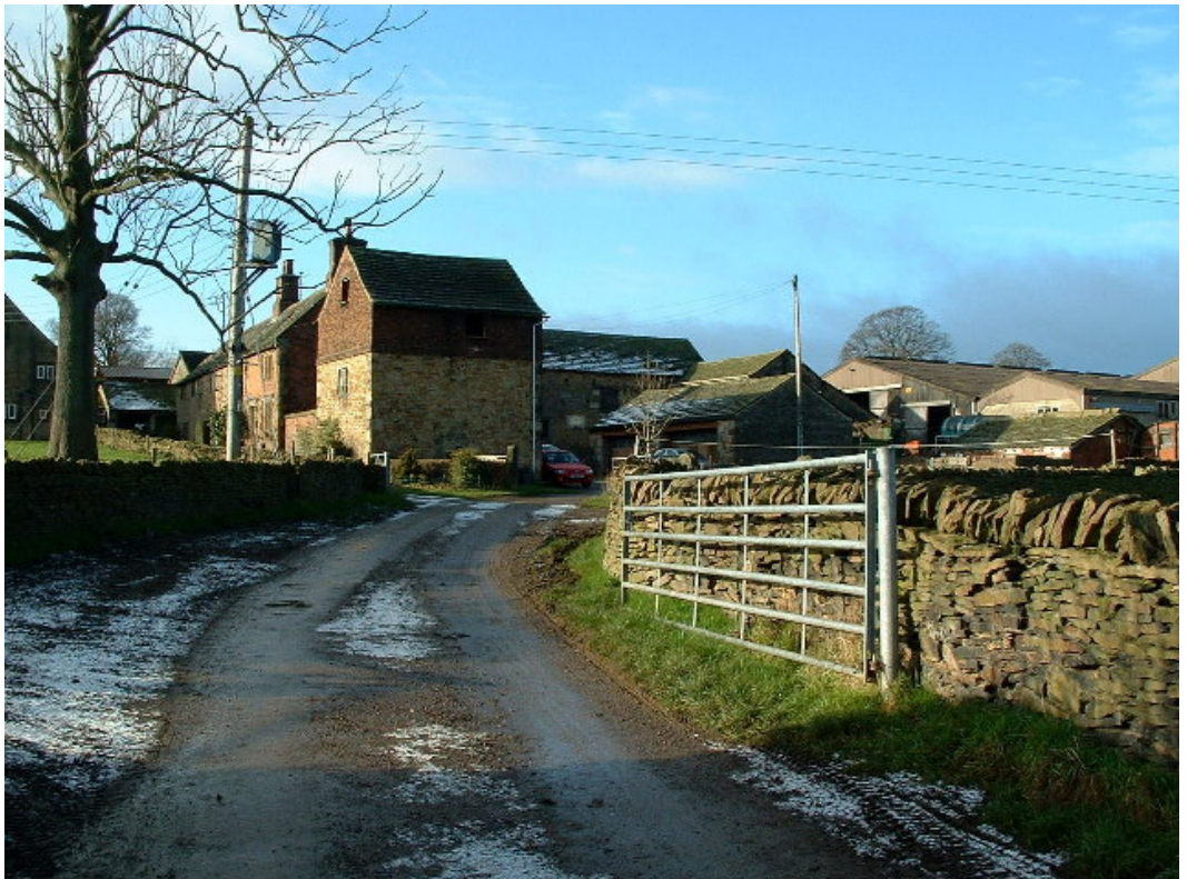
The South gable, and East elevation of the Dovecot, viewed from Jowett House Lane
