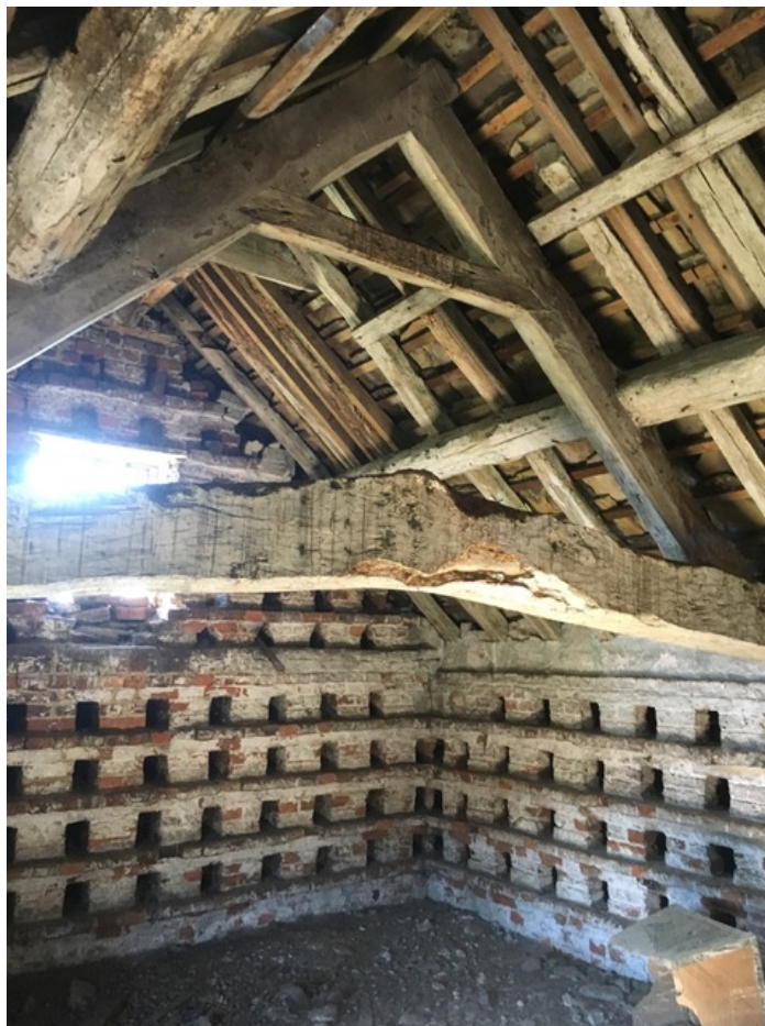
Nesting niches at second floor level, and the original roof truss
