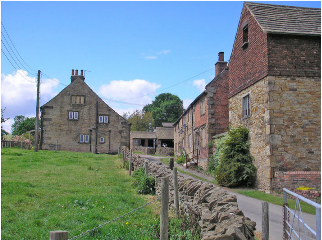
The South gable elevation, with Jowett House Farm beyond
