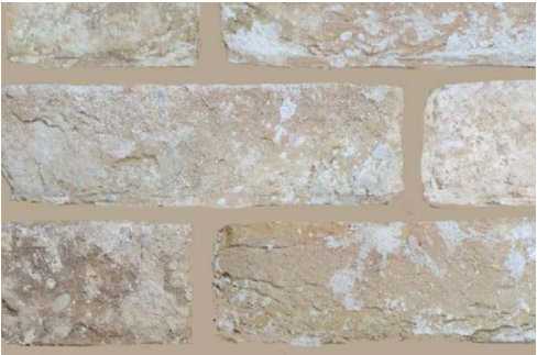
Brickwork infill - Honey / buff multi with matching mortar
