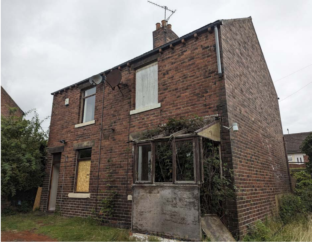
Plate 1: The southern elevation of B1.
