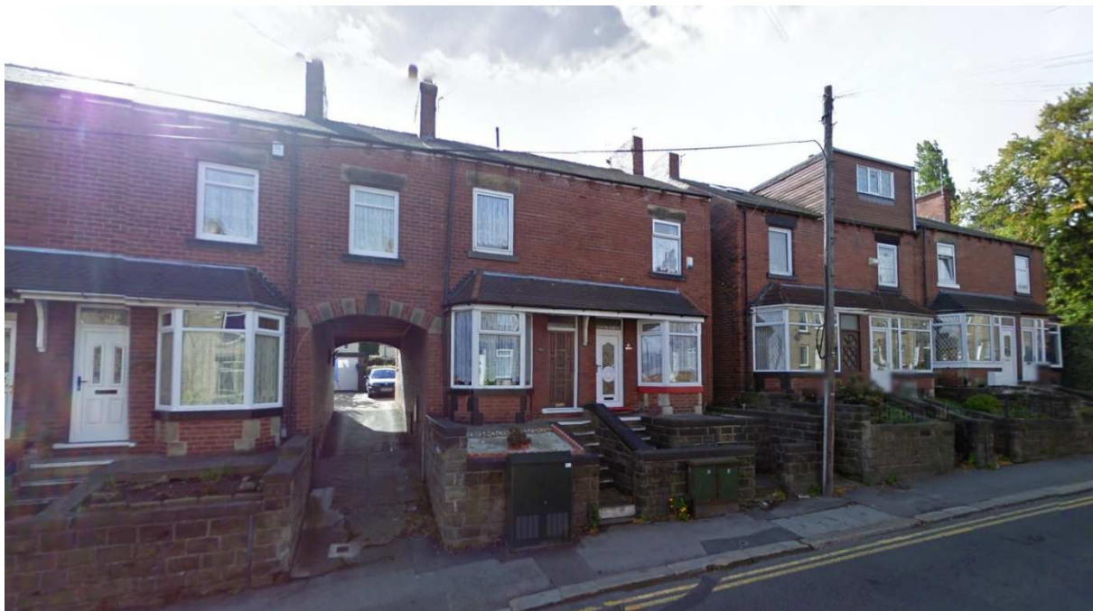
View of existing properties on Hough Lane
