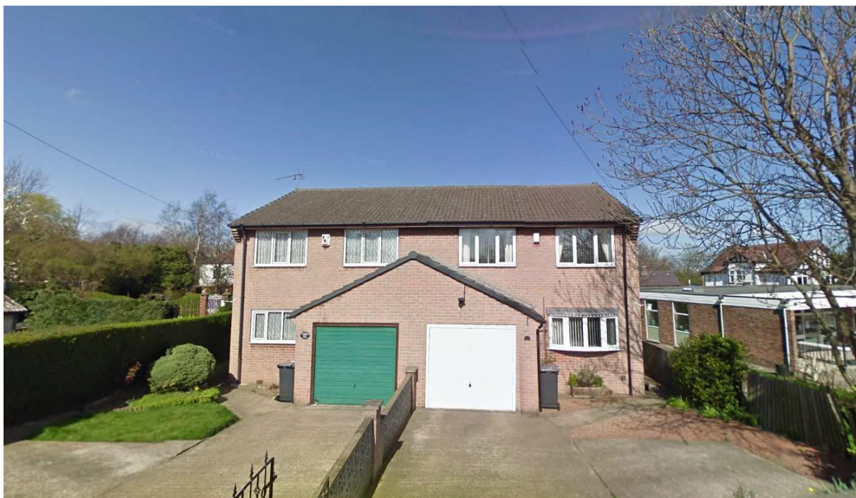
View of existing property on Bondfield Close
