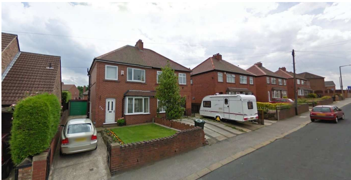
View of existing properties on Summer Lane
