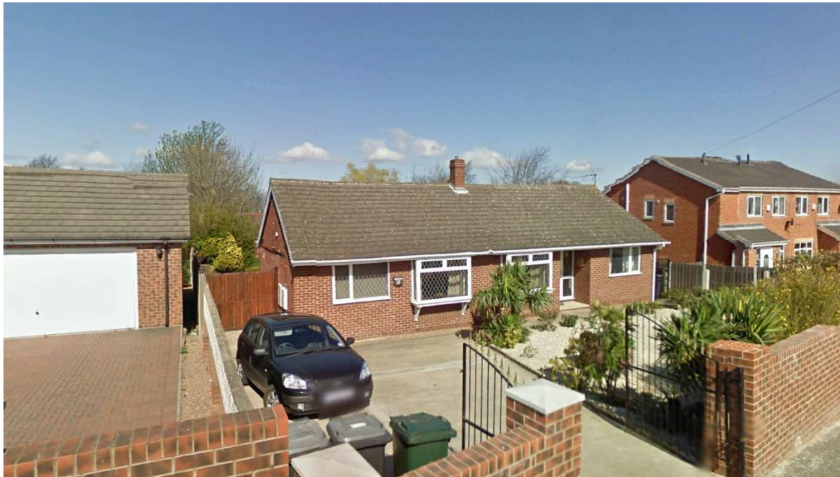
View of existing properties on Bondfield Close
