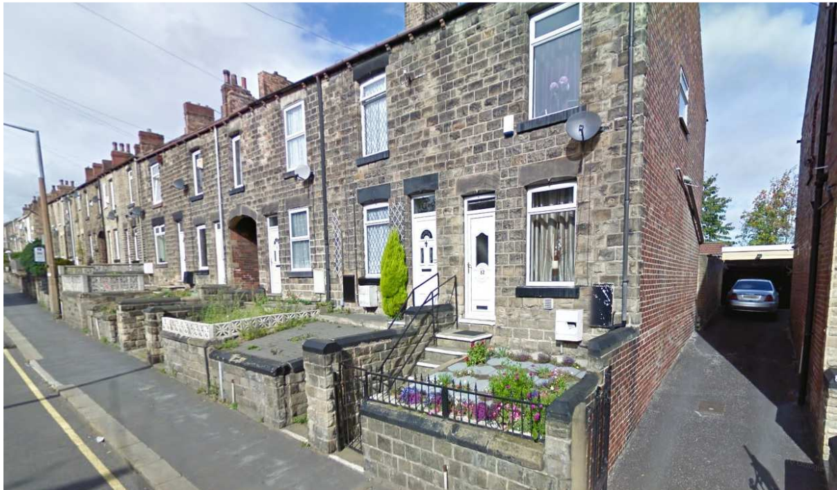
View of existing properties on Hough Lane
