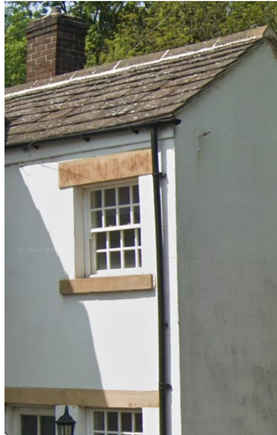
Existing Resin Stone Replica roof tile.
