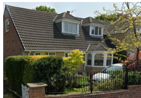
CONCRETE INTERLOCKING TILE- TIVY DALE DRIVE/ CONSERVATION AREA
