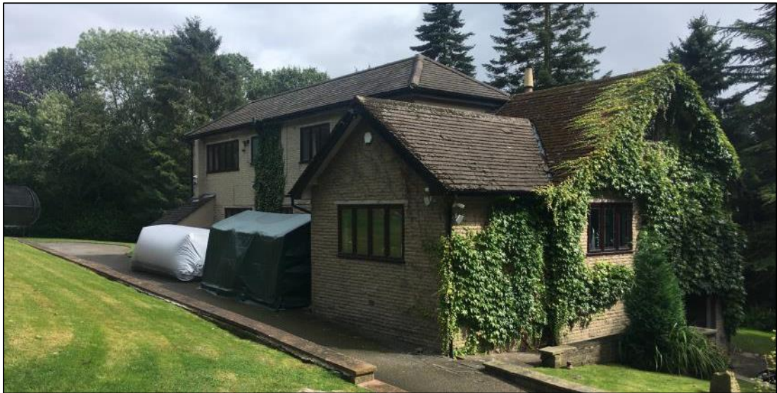
Plate 1. Northwest corner of dwelling
