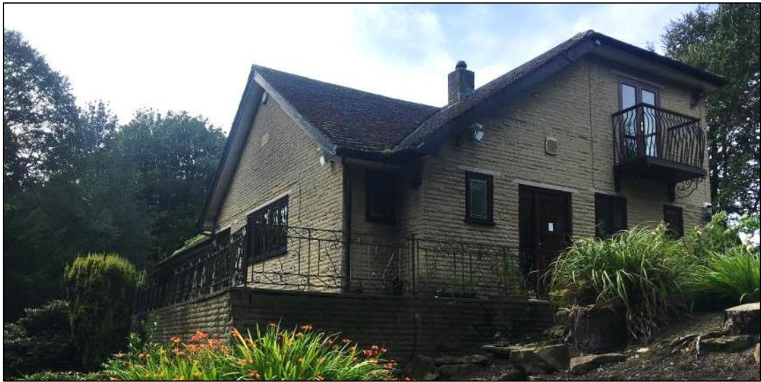
Plate 2. Southeast corner of dwelling
